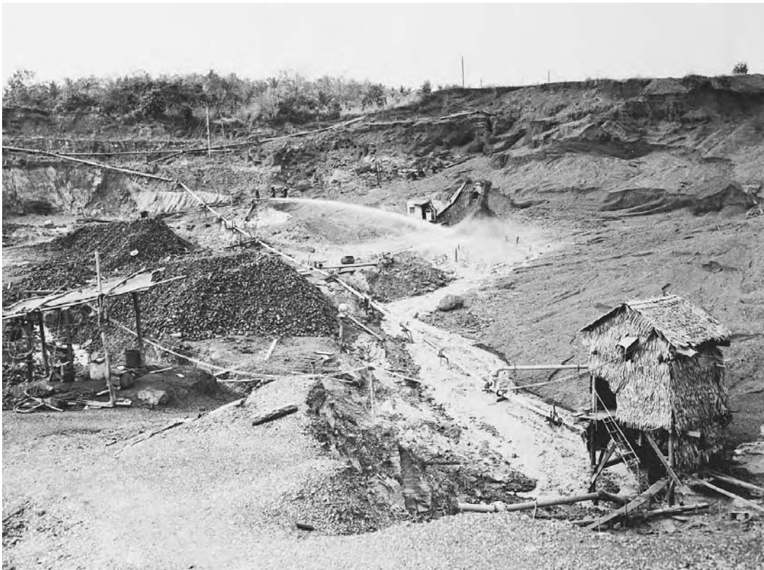
British Malaya once led the world in tin production. Here, at a Chinese tin mine, a primitive work hut and modern mining equipment offer a study in contrast. Water is pumped into a tin-bearing area and tin ore is then sifted from the mud. (Bettmann/Corbis)
