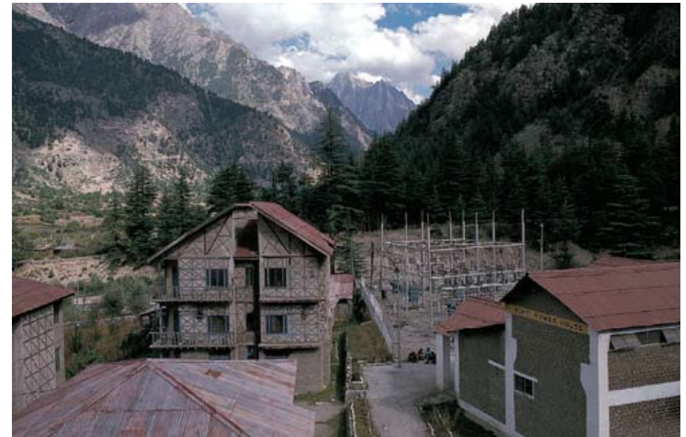
Mini-hydropower scheme in the Sangla Valley provides electricity for local villages.
