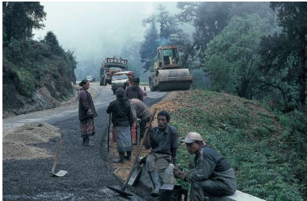
Road workers, Bhutan.
