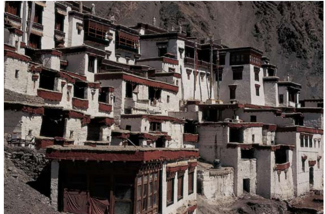
Flat-roofed adobe houses are common in the Tibetan-dominated villages of the arid trans-Himalayan zone.
