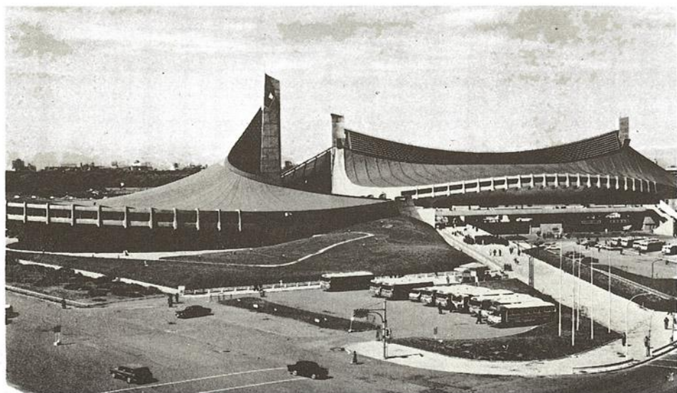
National Indoor Gymnasium, Tokyo. Architect: Tange Kenzō
