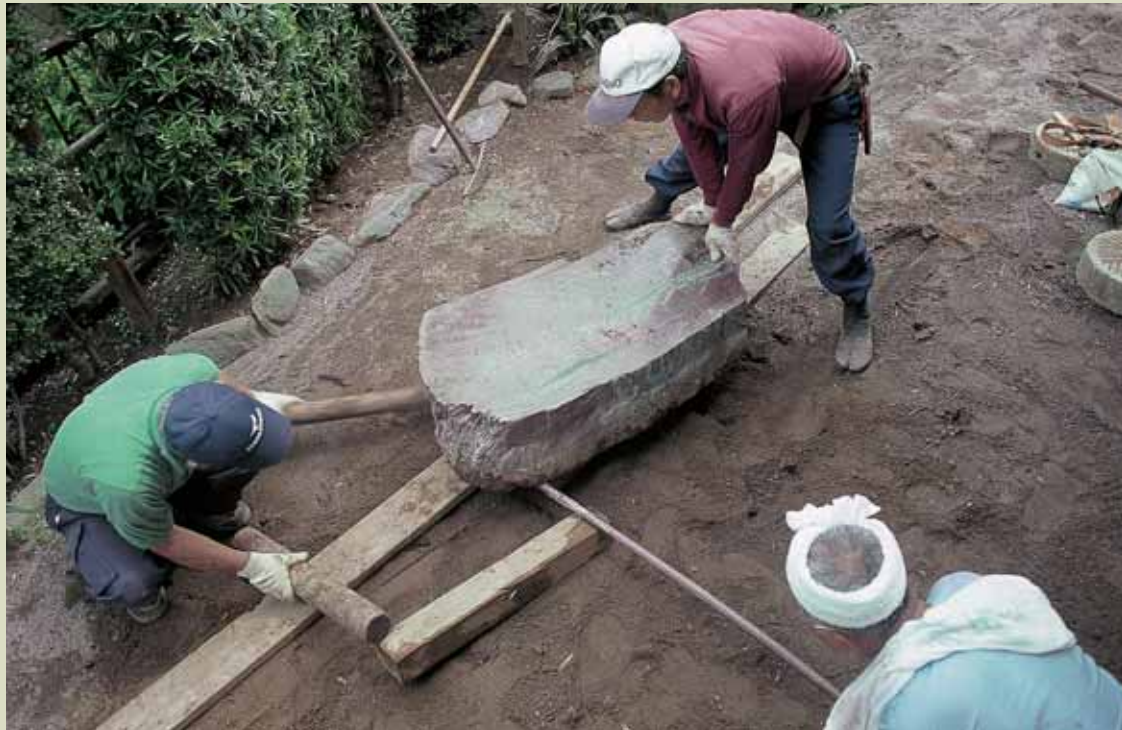
ABOVE Moving a heavy stone in a private garden by traditional methods, using wood rollers, planks and plenty of muscle.
