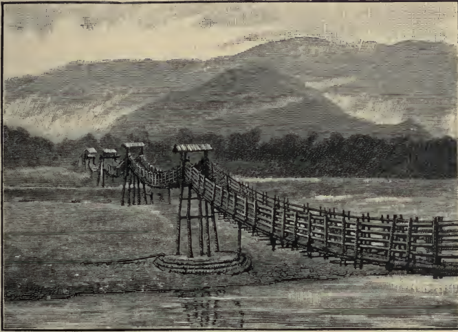
Bridge near Kwan-hsien (Ch'eng-tu).
