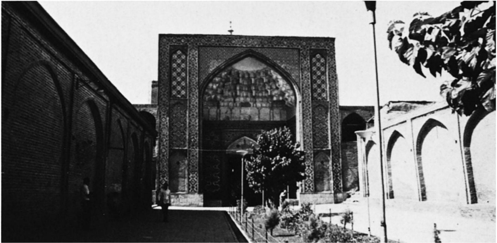
48 (a) Qazvīn, Masjid-i Shāh, 1806. Entrance.
