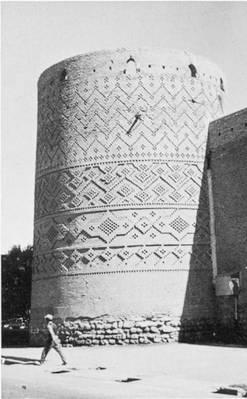
2 (a) A corner of Karīm Khān's arg (citadel) in Shīrāz.
