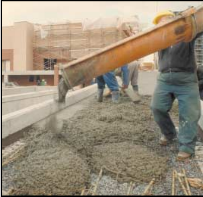
A modern construction crew pours concrete at a building site.
