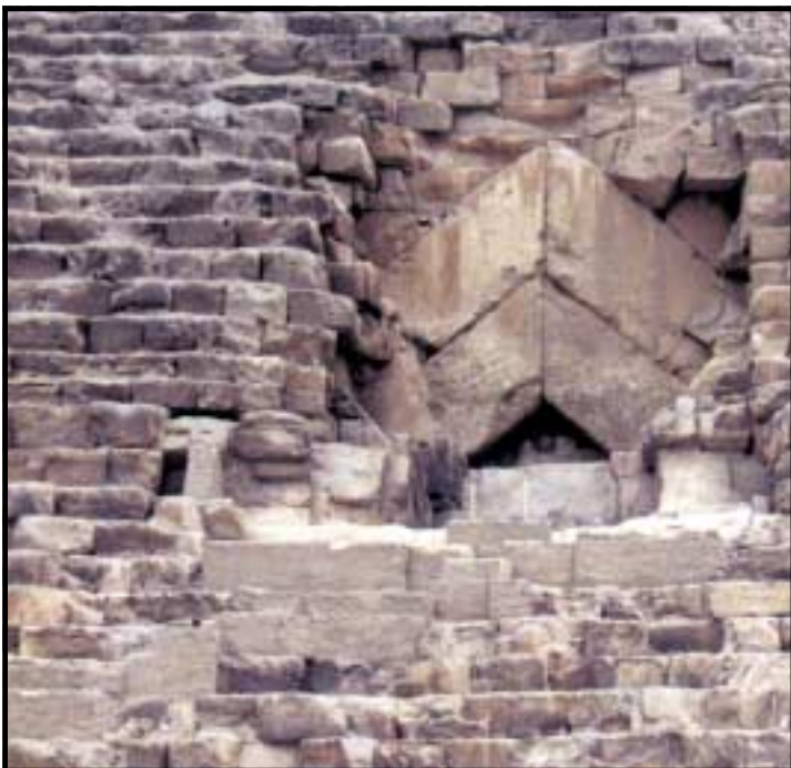
Giant building blocks in the Great Pyramid and elsewhere continue to baffle modern scholars. The angled blocks shown weigh over 40 tons each.
