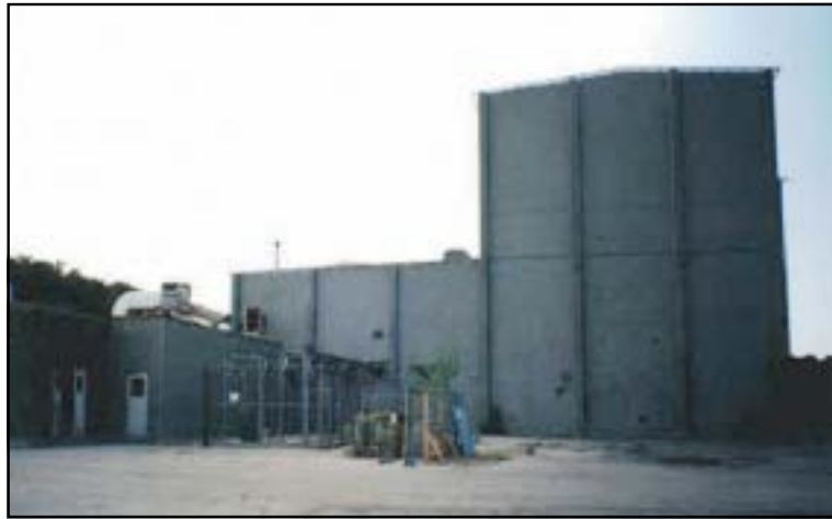
The Former Sodium Reactor Experiment Containment Building at the Santa Susanna Site
