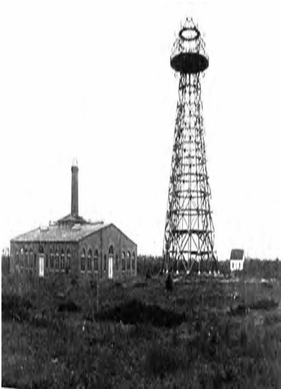
The tower and power station partially built at Wardencllyffe, Long Island.
