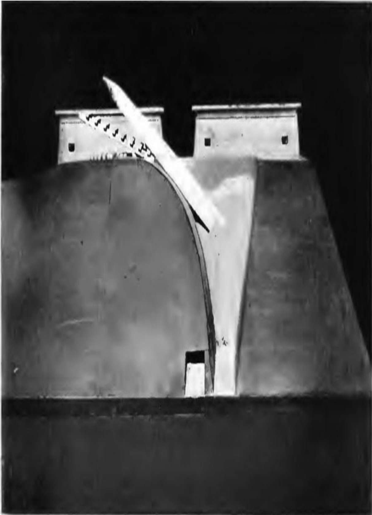
Engelbach's sectional model with the obelisk in the tunnel while sand is removed.
