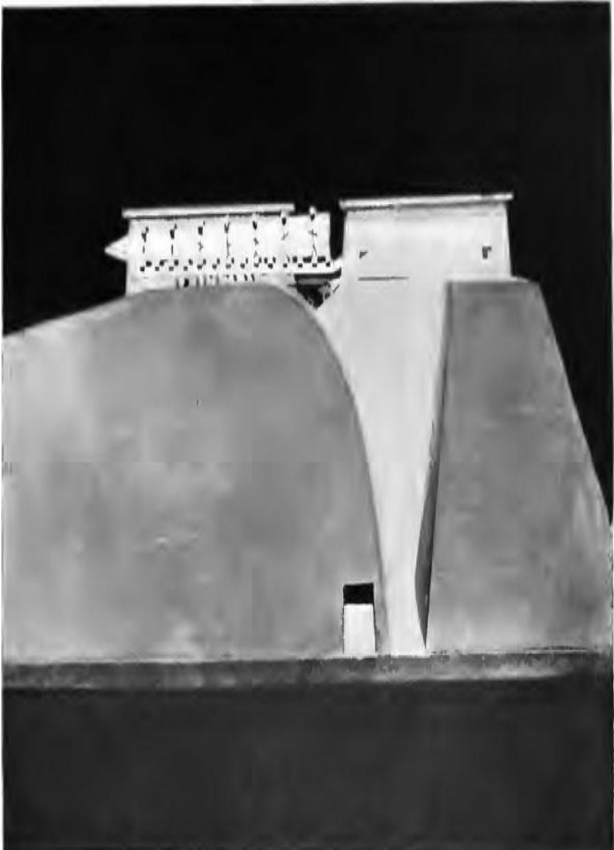
Engelbach's sectional model with the obelisk overhanging the sand tunnel.
