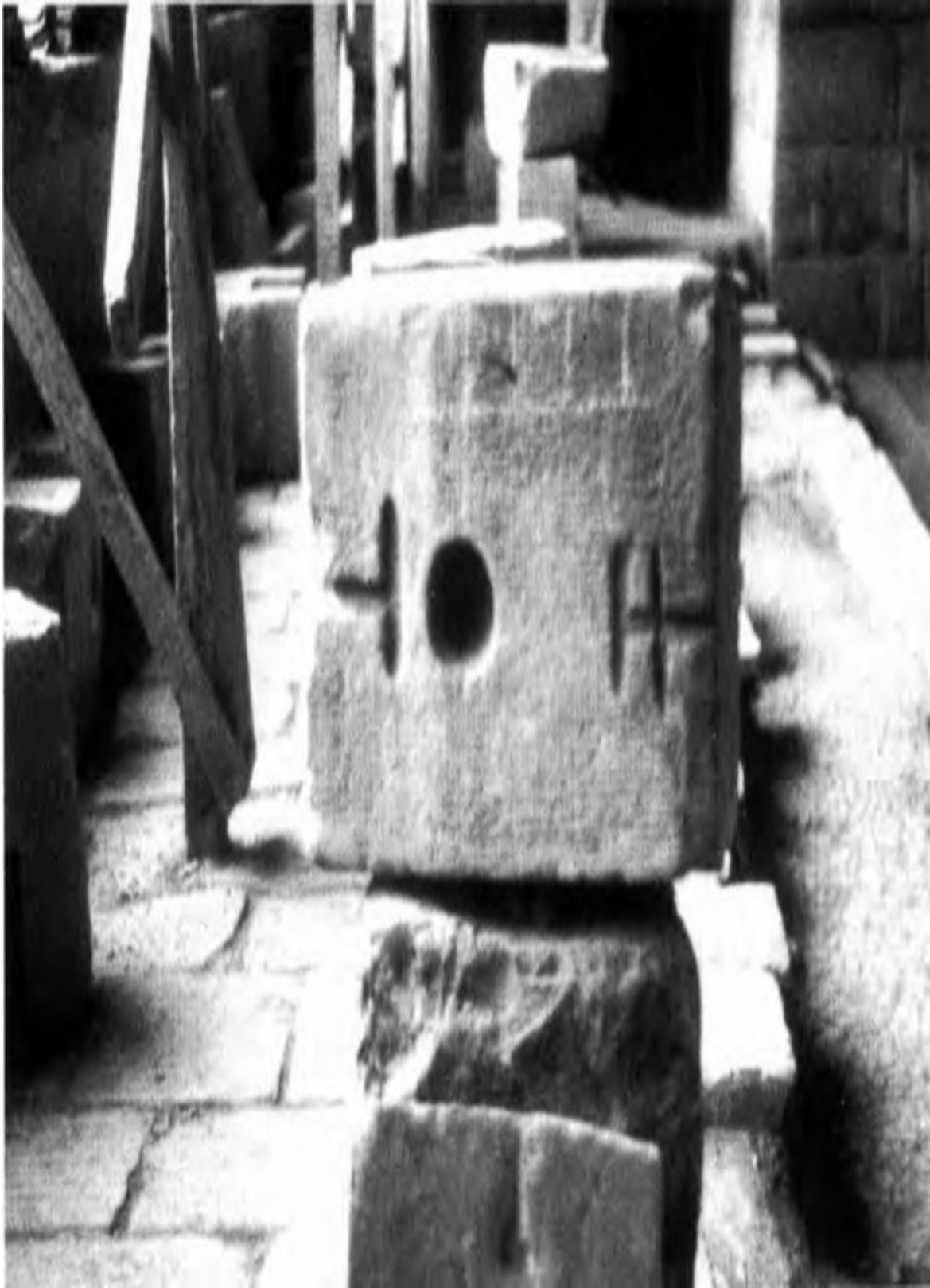
A photo from Protzen of some of the keystone cuts on blocks in Cuzco.
