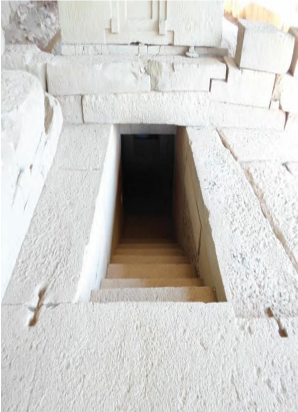
Keystone cuts for metal clamps can be seen on ancient structures at Axum, just like in Egypt;
