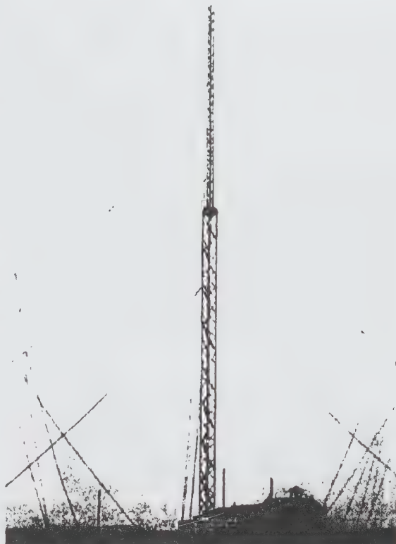
One of Marconi's wireless towers which resembled Telefunken's towers at Tuckertown, NJ and Sayville, NY. Credit: MetaScience Foundation
