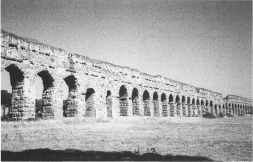
Figure 3.1 Remains of the Aqua Marcia outside Rome. The majority of most Roman aqueducts were underground, but some portions were carried on above ground arcades such as these.
