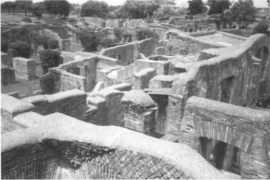
Figure Appendix IV.1 View of ruins in Ostia showing brick-faced construction technique.
