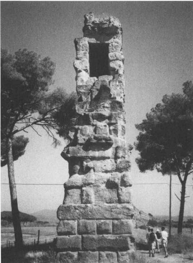
Figure 3.3 Cross-section of aqueduct showing the covered channel through which the water flowed.
