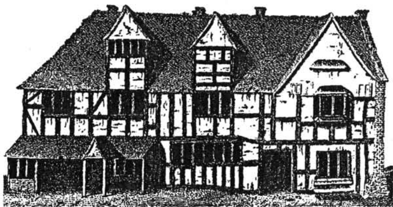
Shakespeare's house: a classic example of timber-framed construction. [Gentleman]
