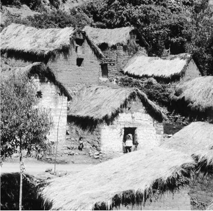
Homes constructed of adobe and thatch in modern Ecuador, a style of housing that has been in use in some areas of Latin America for hundreds of years. (The Art Archive / Gianni Dagli Orti)
