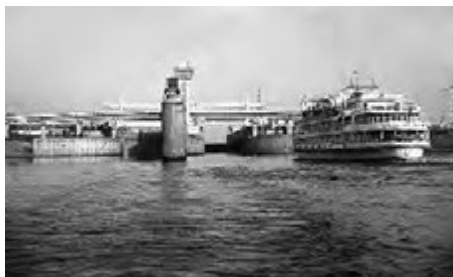
Fig. 191. Lock at the kanal Moscow – Volga river
