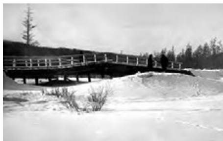
Fig. 146. Hazard of aufeis: Destruction of a bridge by the river aufeis at a tributary of Amur river
