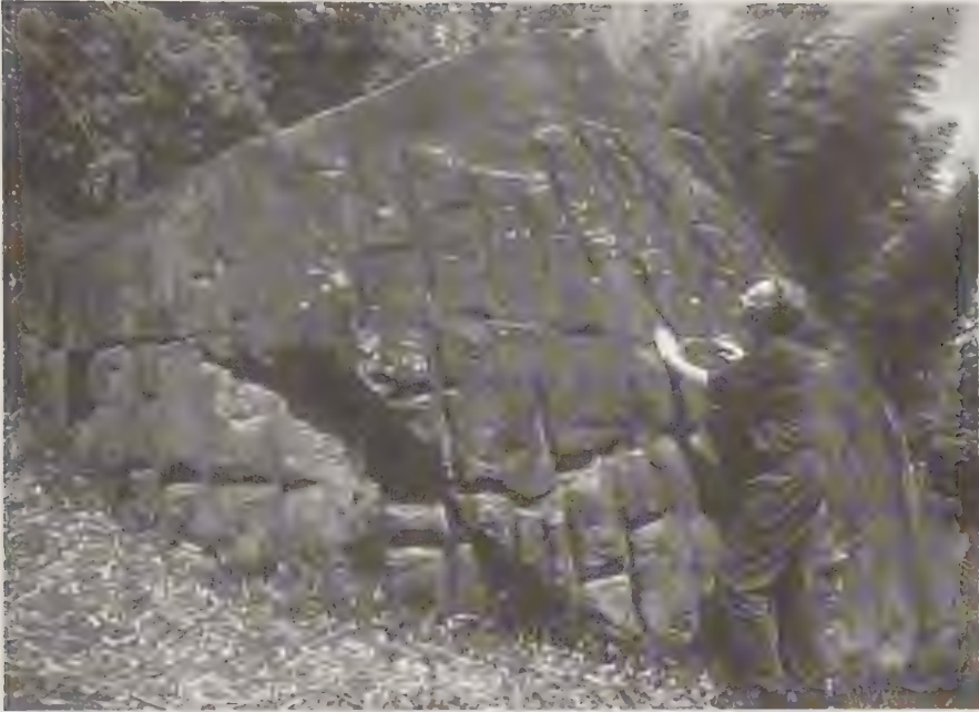
Above ground markings at Masada no Iwasure
