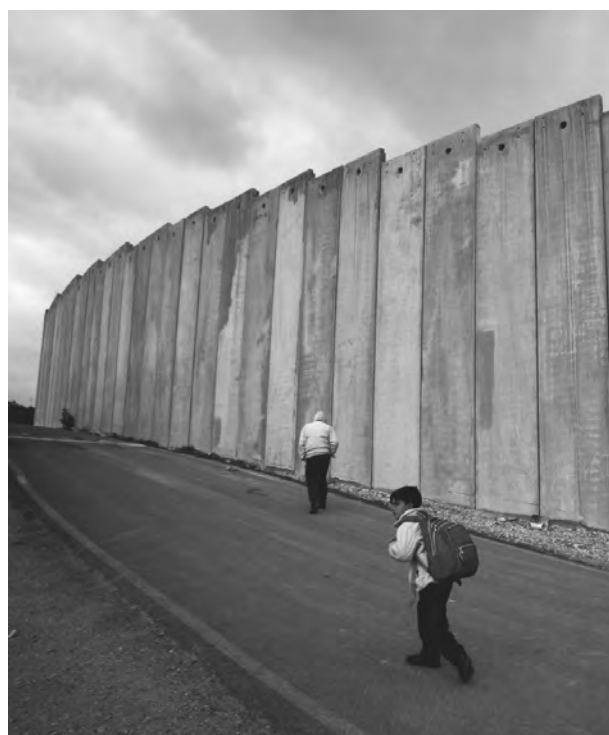
Palestinians Walk Past Israel's Controversial Separation Barrier in Jerusalem, 2007. In 2002 the Israeli government, citing the need to maintain internal security, began building a thirty-foot-high concrete-and-barbed-wire Separation Barrier throughout historic Palestine. AP IMAGES.
