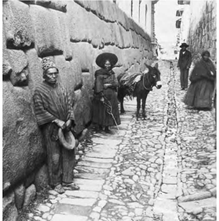
Peruvians surrounded by the mortarless masonry of the ancient Incas, in Cuzco, Peru
