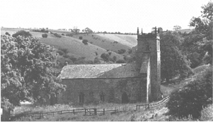
52 Wharram Percy Church, Yorkshire, showing the blocked arcading of the thirteenth-century north aisle, demolished in the later Middle Ages (R.C.H.M.)
