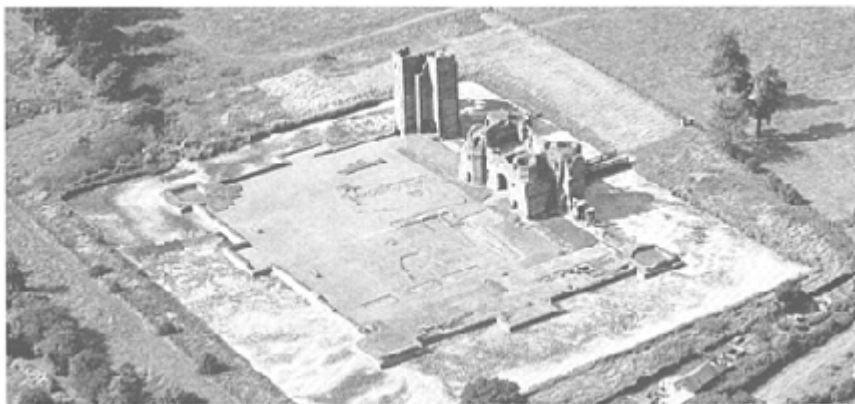
123 Symmetrical planning at Lord Hastings's unfinished late-fifteenth-century castle at Kirby Muxloe, Leicestershire (Aerofilms)
