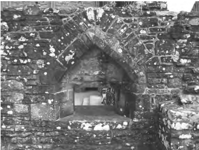
4. Serving hatch. Tintern Abbey kitchens, Monmouthshire
