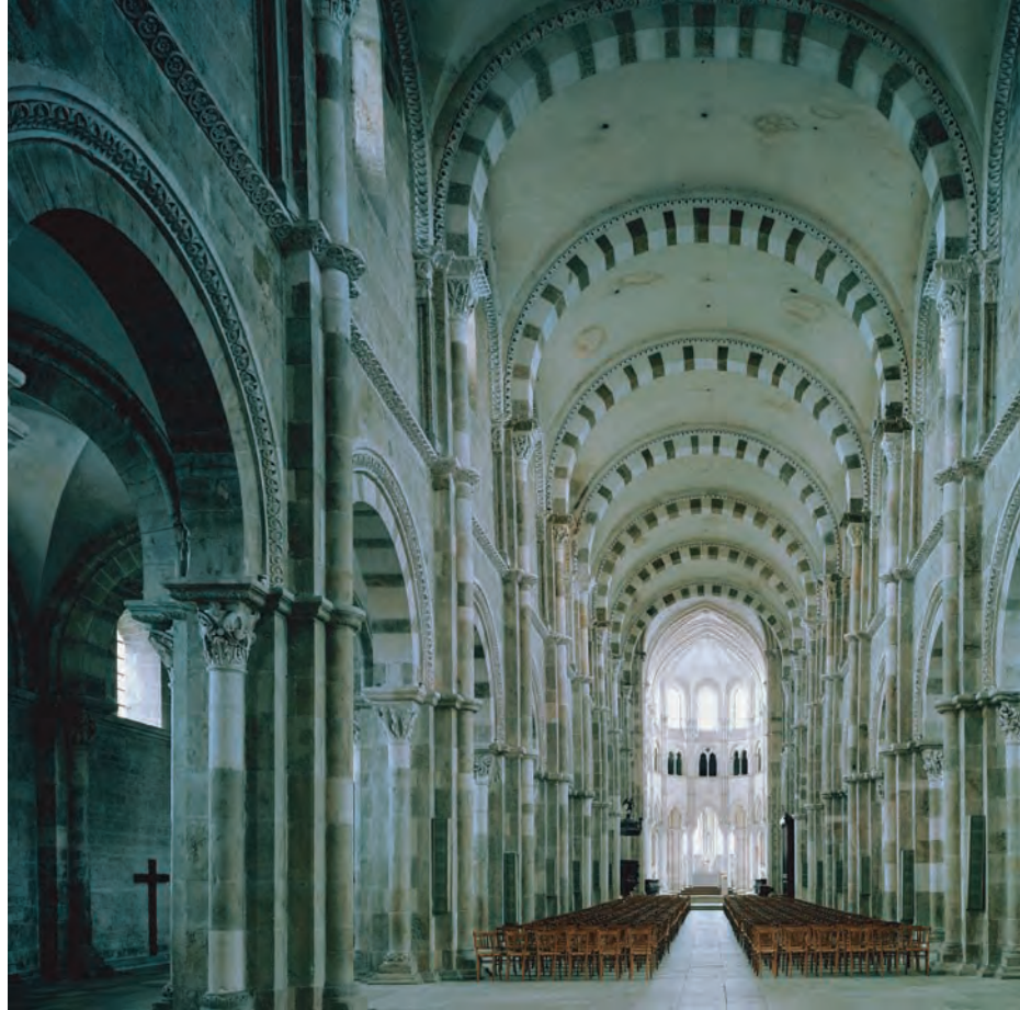
Above: This French church has a classic Romanesque barrel-vault roof.
