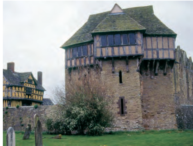
Top: Stokesay's north end, with the lord's private apartments on top, surrounding wall, and the later timber-framed gatehouse (built in the 17th century). The great hall, seen here ( center ) from the east, links the private apartments to the tower keep, with its separate entrance.
