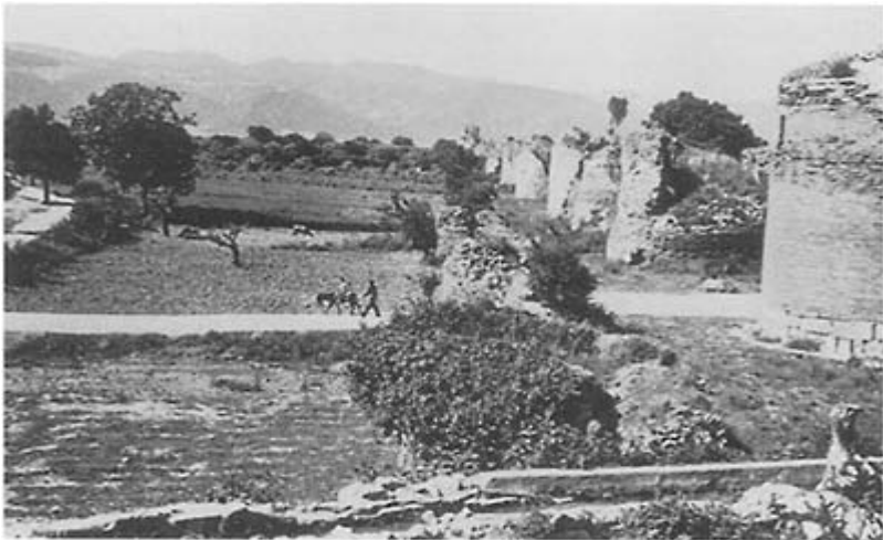
Ill. 55 The defensive walls and bastions of Roman/Byzantine Nicaea at the north-east end of town, with fertile fields in the foreground and the mountains of Bithynia in the distance.
