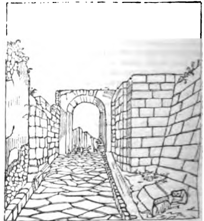
The centre of the way was a little elevated, so as to permit the water to run off easily, and hence
