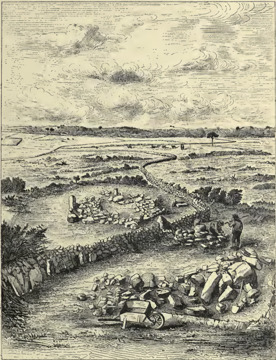
PRIMITIVE CONSTRUCTIONS NEAR THE WINDMILL OF KERMAUX.
