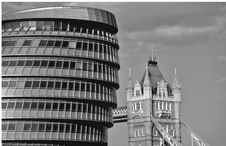
Britain, past and future—the innovative Greater London Authority Building, whose bulbous shape is designed to control energy use, and the Tower Bridge (Neil Setchfield/Lonely Planet)
