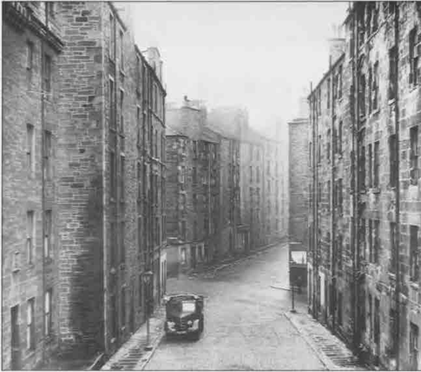
13 Typical Edinburgh tenements, built in the 1860s: a dense, high-rise form of residence which was unusual in England.
