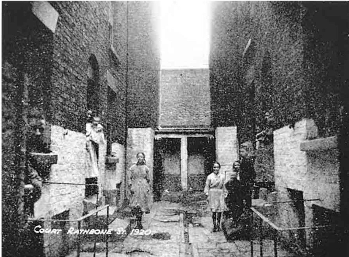
11 Nineteenth-century court housing in central Liverpool, photographed in 1920, showing the congestion and lack of through ventilation.
