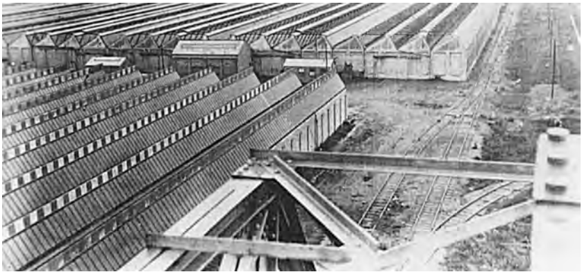
23 Slough Estates Ltd: the trading estate in the late 1920s, showing standard factory units leased to firms.
