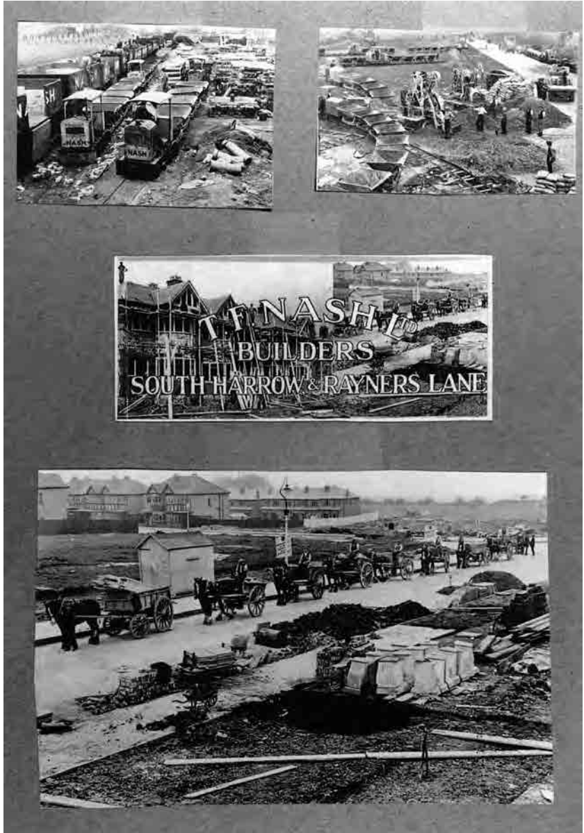
19 Large-scale construction of speculative houses by T. F. Nash Ltd in 1932. The firm owned a farm of 250 acres near Rayner's Lane station on the Metropolitan Line. From A. A. Jackson, Semi-Detached London (London, 1973).
