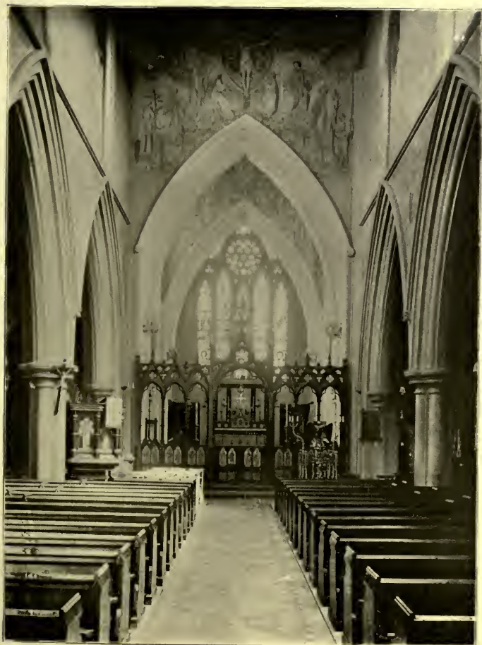
ST. MATTHIAS', STOKE NEWINGTON. Interior, looking East.
