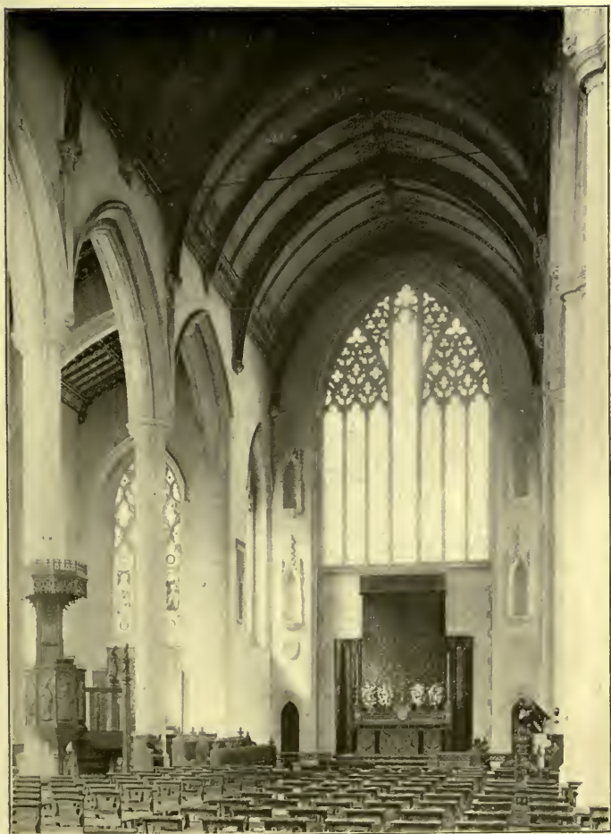
HOLY TRINITY, KENSINGTON GORE. Interior, looking East.
