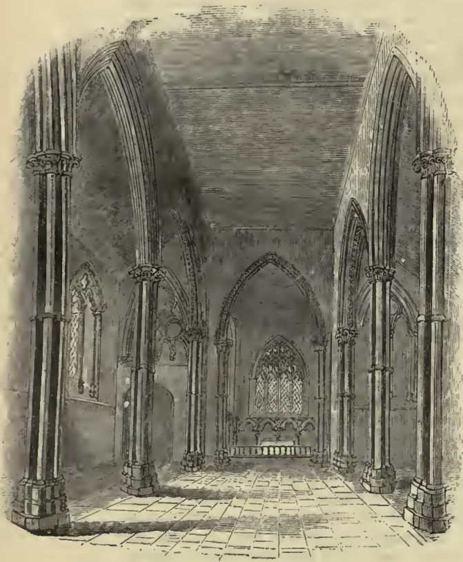
1047.—Stone Church: Nave and Chancel
