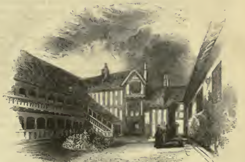
1546.—Leicester's Hospital, Warwick.
