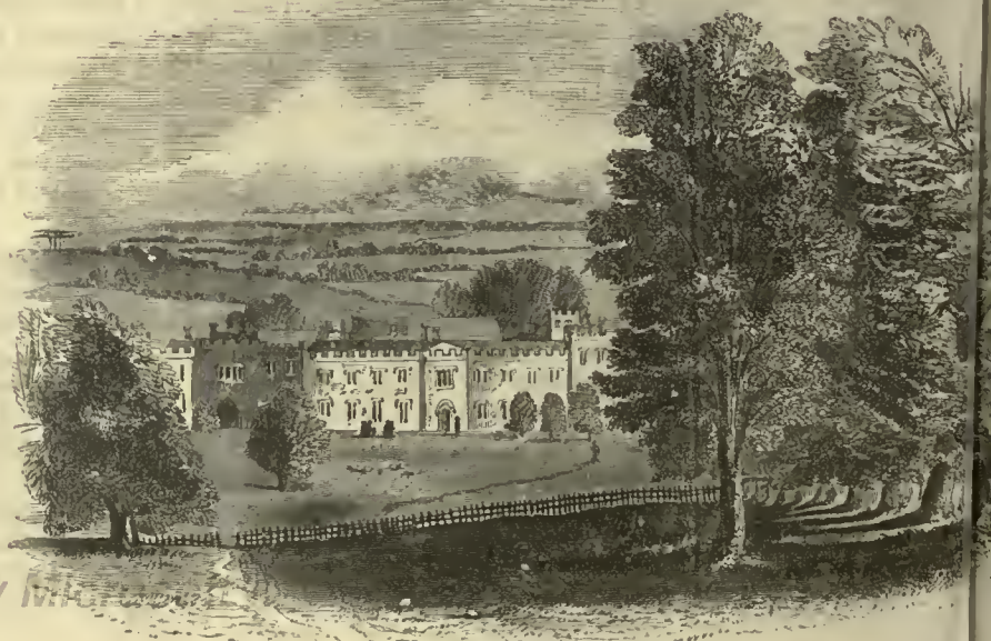
1552.—Penshurst. General View.
