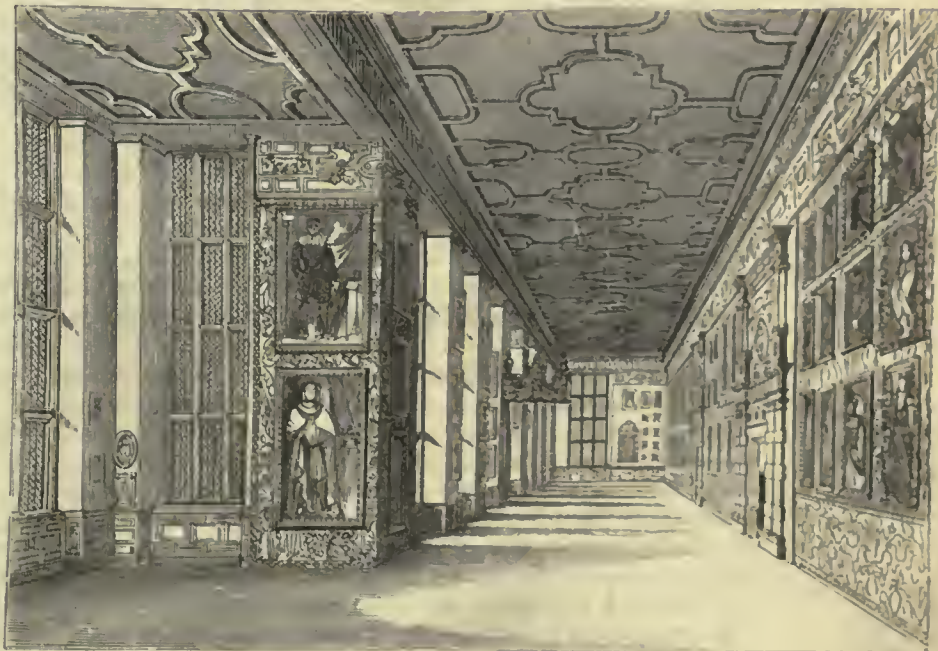
1670.—Hardwick Hall, Derbyshire.
