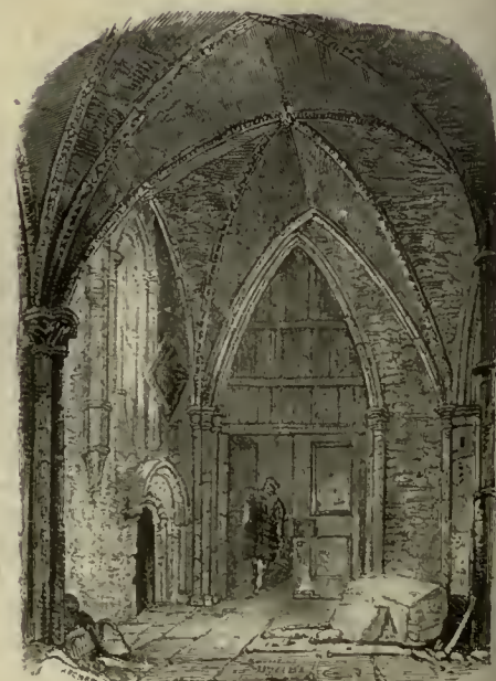
546.—Norman Arch, St. Mary Overies.
