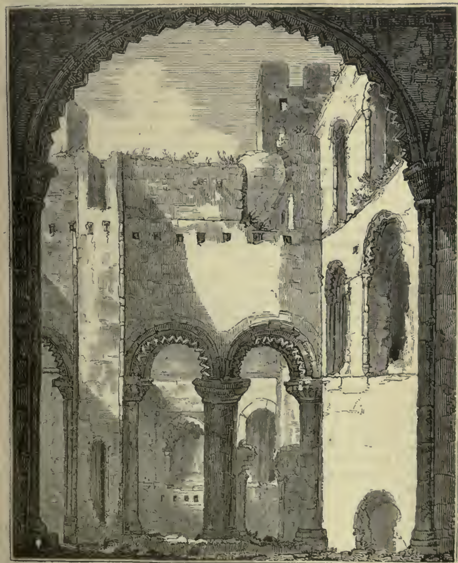
373.—Interior of the Remains of the Upper Story of Rochester Castle.
