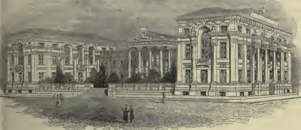
2272.—Taylor Institute, Oxford, erected 1844.
