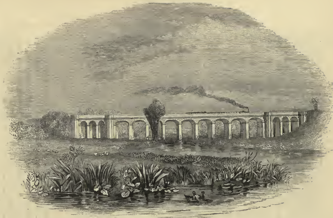
2462.—Viaduct over the Upper Avon.
