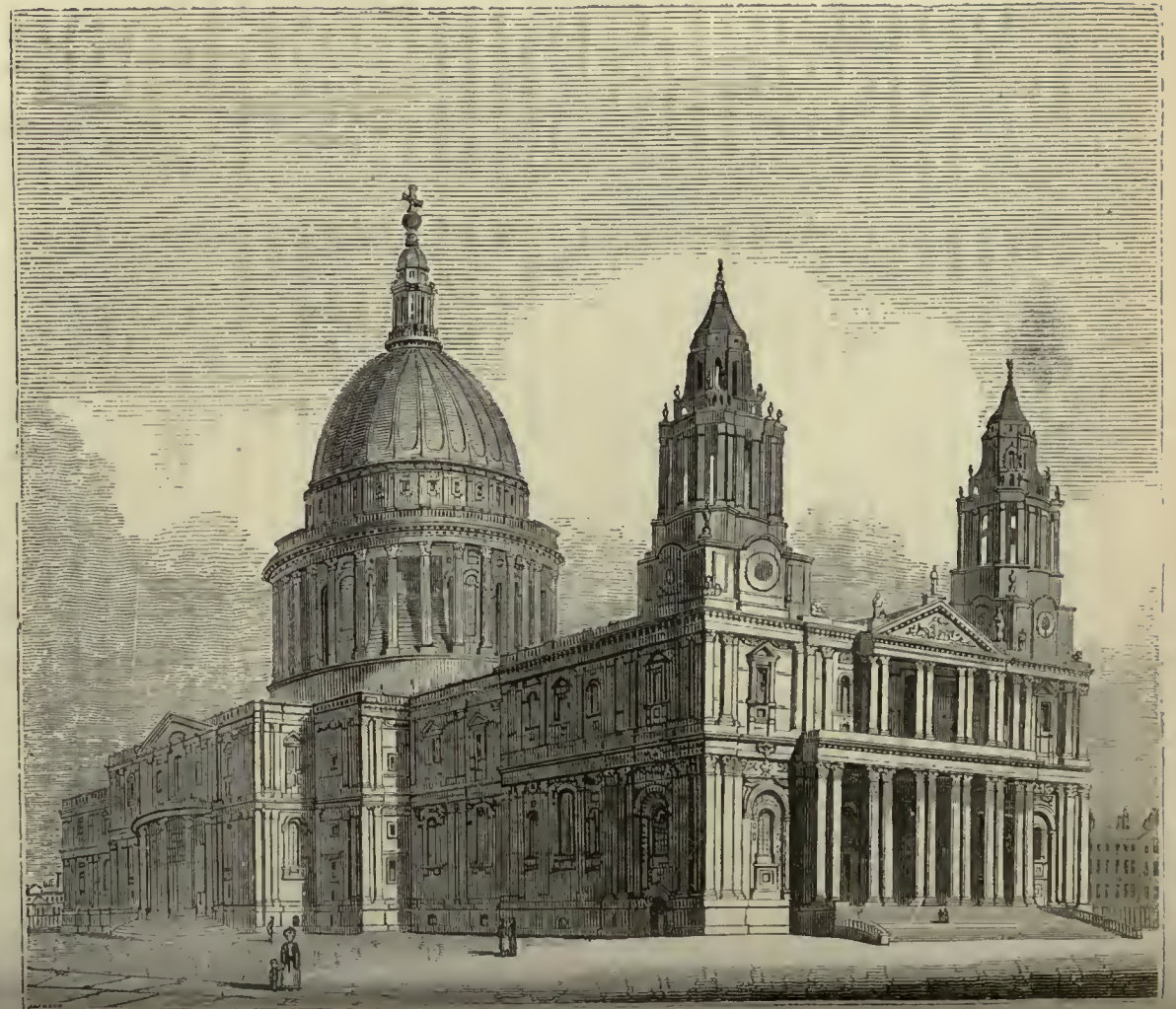
2020.—Northwest View of St Paul's Cathedral.
