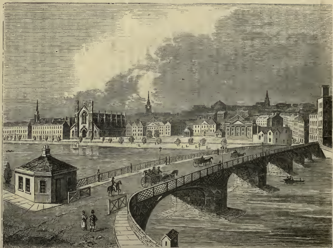
2505.—StocKwell Bridge, Glasgow.
