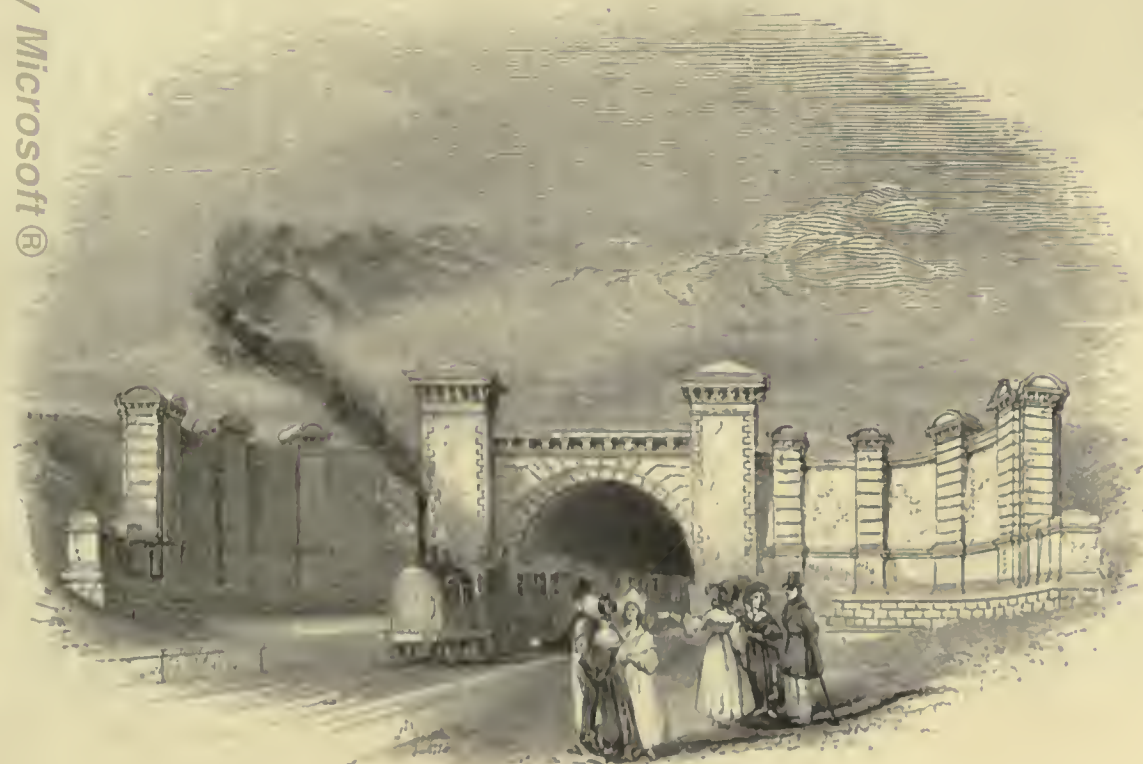
2461.—Fyfe's Hill Tunnel.
