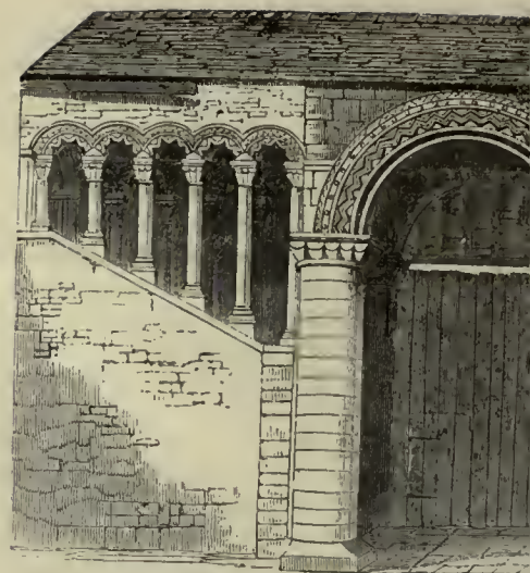
569.—Staircase in the Conventual Buildings, Canterbury.
