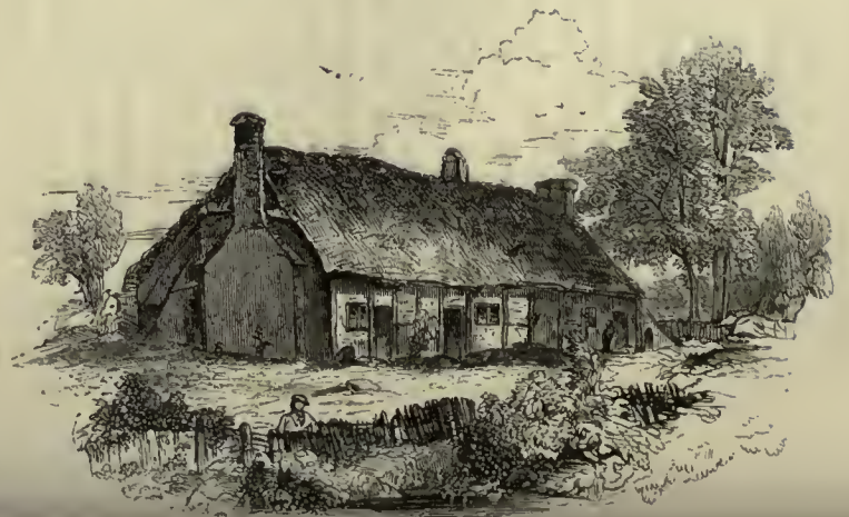
2035.—Butler's House, Pershore
