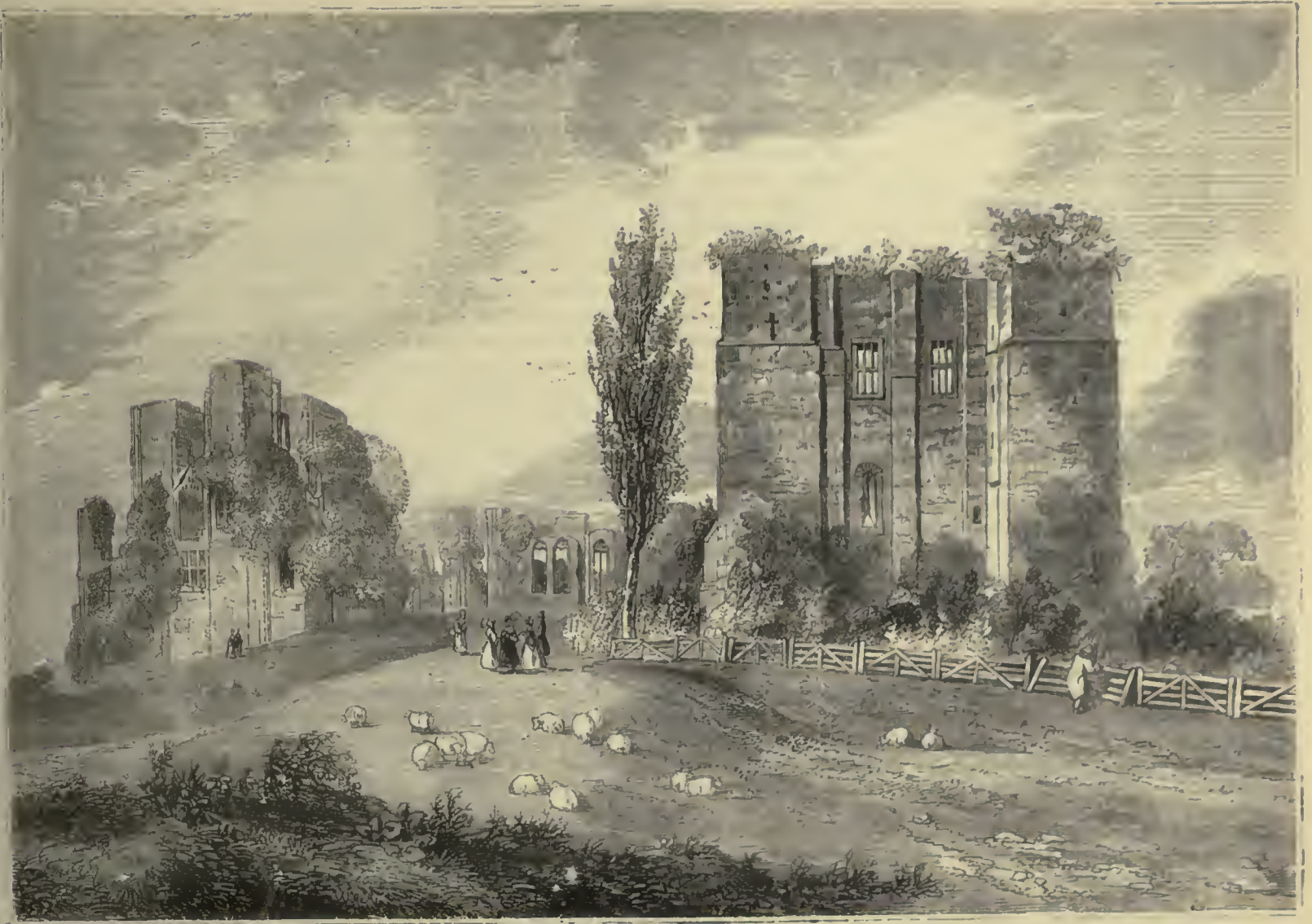
822. View of Kenilworth Castle from the Gate-House
