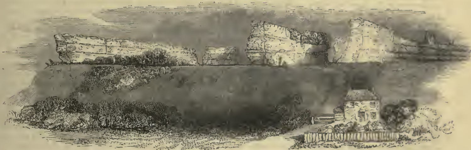
99.—Richborough. General View, from the East.
