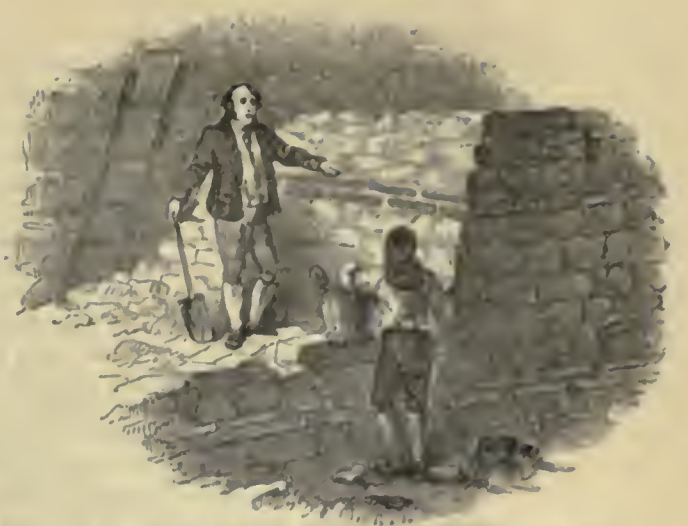
149.—Part of the Roman Wall of London excavated behind the Minories.
