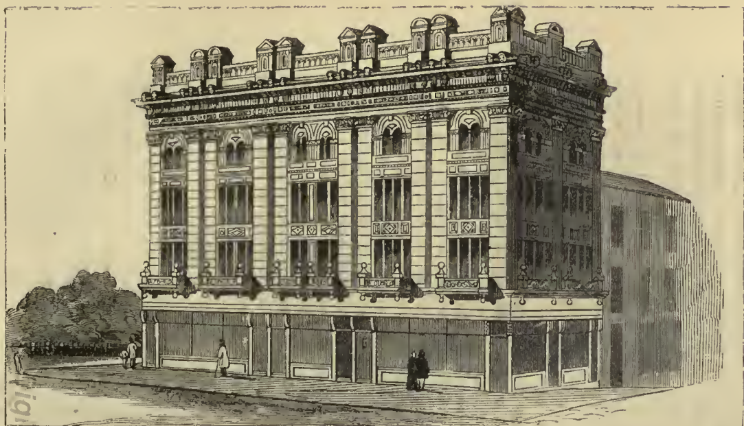
2506.—Buildings in Leicester Square
