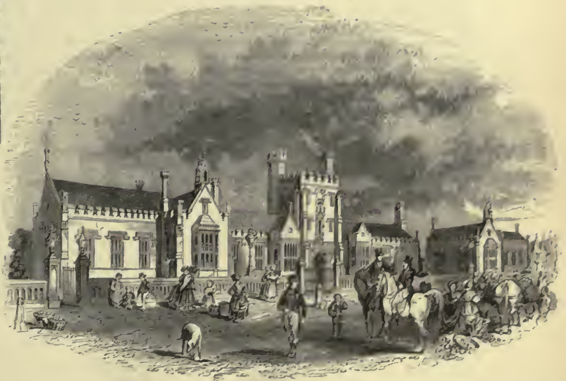
2287.—Bedford School (as rebuilt).
