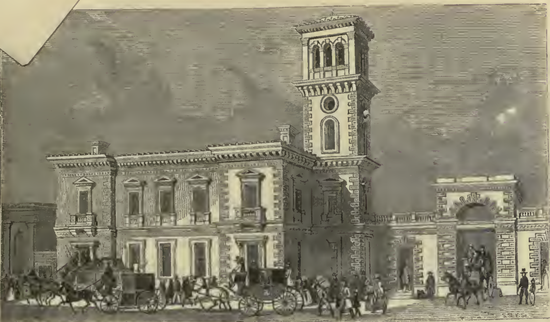
2464.—London Bridge Railway Station.
