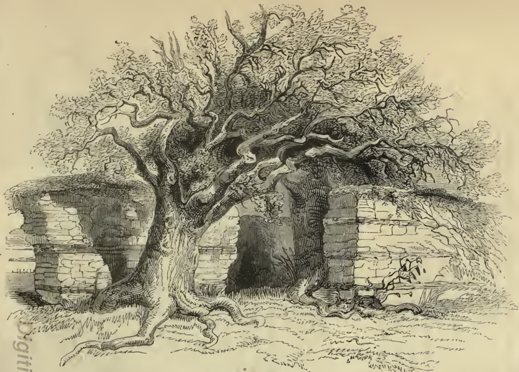
124.—Silchester. The North Wall.
