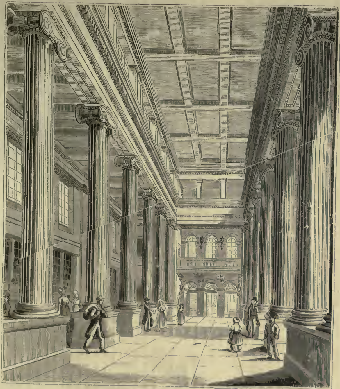
2182.—Hall of General Post-Office.
