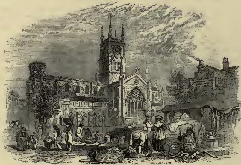
545.—General View of St. Mary Overies, from the South.
