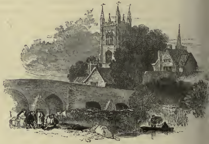
819.—Bridge at Evesham.
