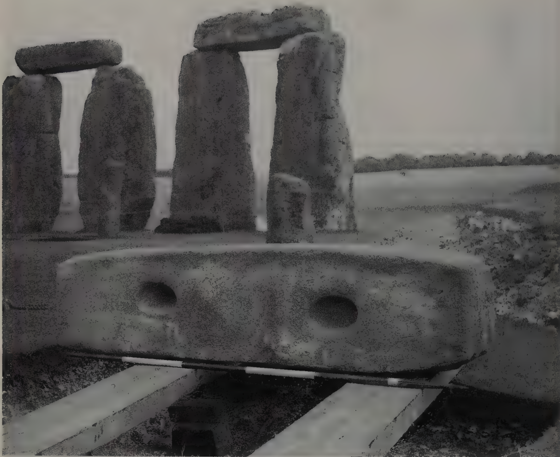
176 (above) The lifting of bluestone lintel no. 36, in 1954, showed its full beauty, and the feeling for shape and form its makers must have possessed. By the left-hand mortice is an oval depression to match the top of its upright.
