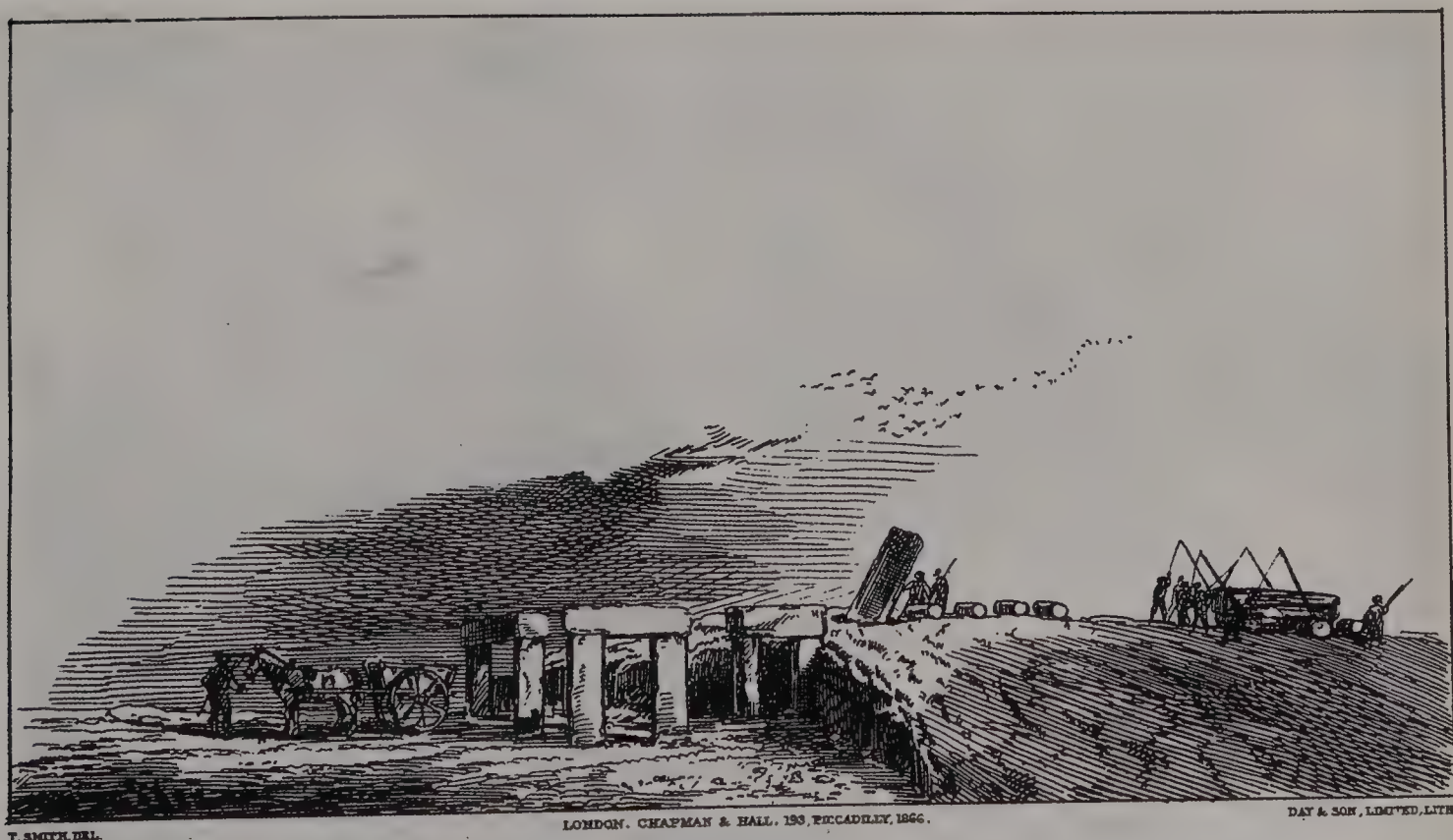
TO REPRESENT THE FORMATION OF STONEHENGE, ONE HALF OF THE MOUND OF EARTH REMOVED, ALSO ONE STONE DROPPING INTO A HOLE AND TIPPING UP FROM OFF THE ROLLERS - ALSO MODE OF CONVEYANCE.
