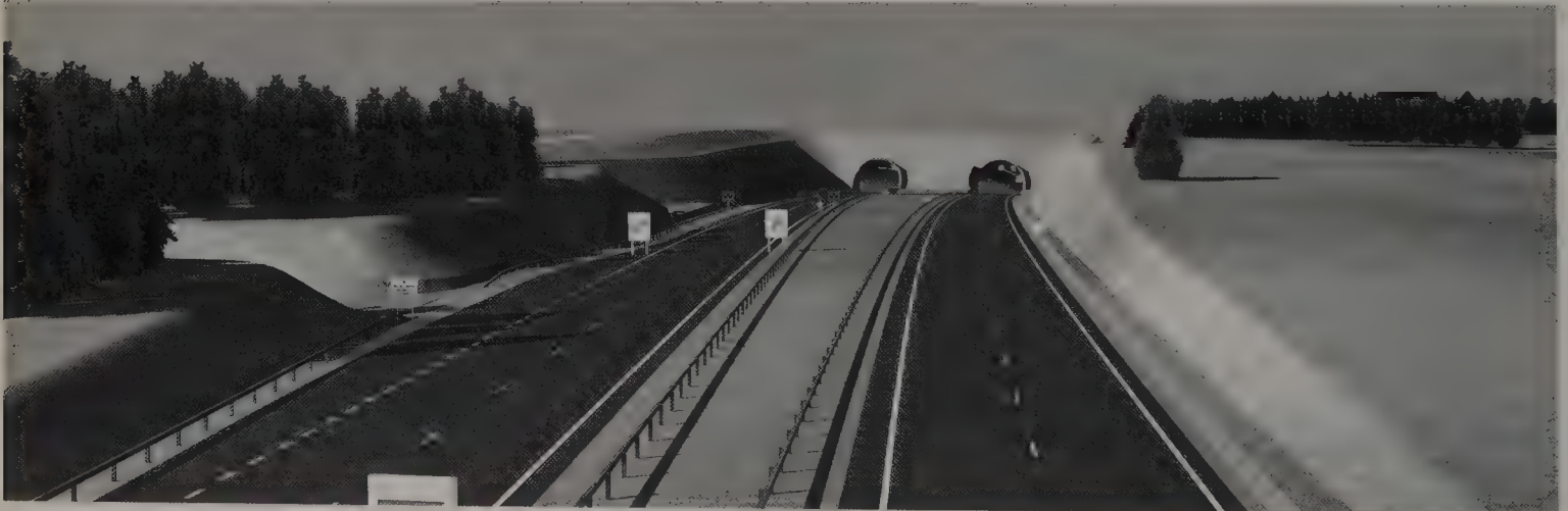
254 The short bored tunnel hides the A303 as it goes past Stonehenge, but the landscape impact of the broad and deep approach cuttings is very substantial, as this image shows.
