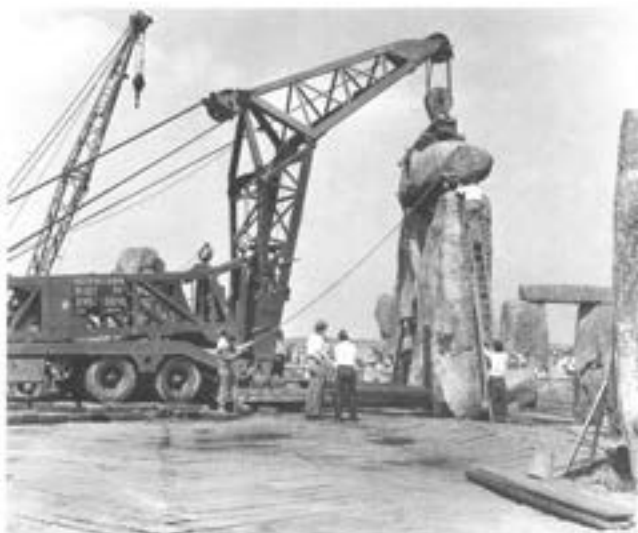
Fig 190 Re-erection of lintel 158 by the 'Brabazon Crane' in 1958 (P50216).
