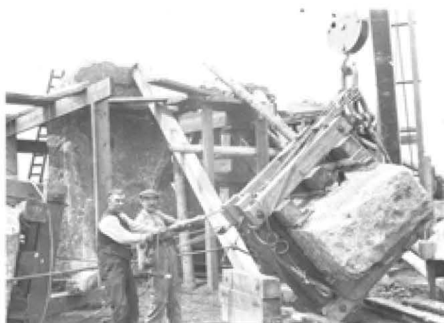
Fig 189 Restoration of the north-eastern arc of the Sarsen Circle in 1920 (Hawley archive)
