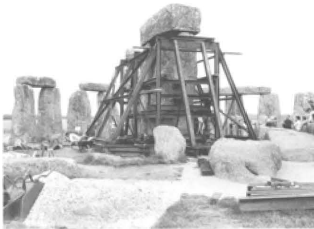
Fig 10 Straightening of Trilithon 53/54 in 1964 following excavation of C56 (P50934)
