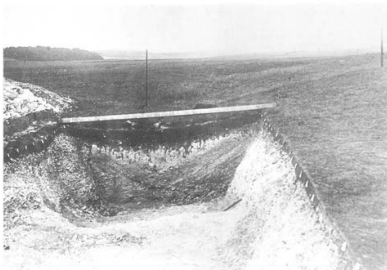
Looking south from Segment 2 into Segment 3 at southern end of C22
