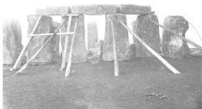
Fig 5 Stones 29–2 propped by wooden poles in 1919 (Hawley archive)
