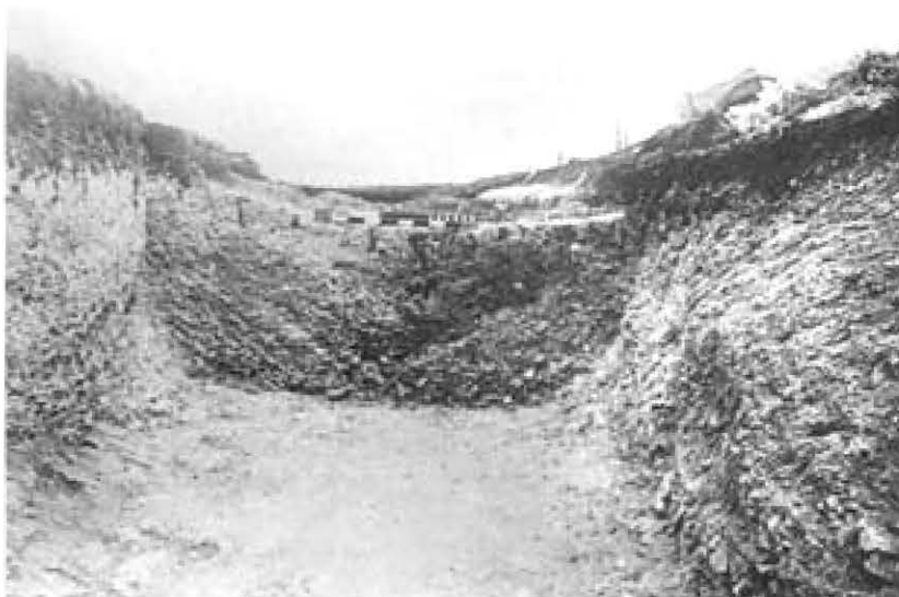
Section within Segment 13 looking east
