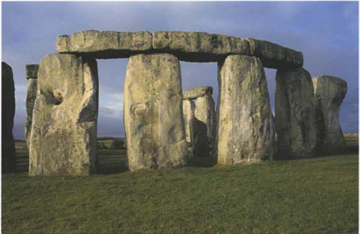
Plate 4.1. The Sarsen Circle (Stone 2 far left): the vertical stones taper upwards, the lintels are curved to form the circle. Notice how closely they fit together
