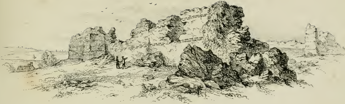
N. W. VIEW OF RICHBOROUGH CASTLE, KENT.
