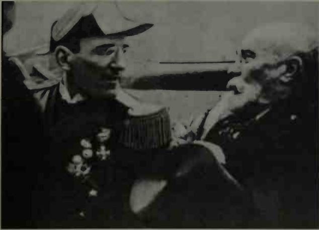
King Alexander with the French foreign minister, Louis Barthou, in Marseilles, France, moments before they are assassinated on October 9, 1934
