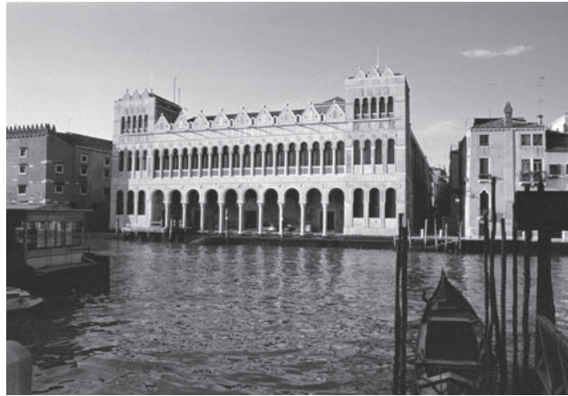
Figure 21.3 Fondaco dei Turchi on the Grand Canal, Venice (now the Museum of Natural History), façade, late twelfth century, restored nineteenth century/ © Sarah Quill/Venice Picture Library/The Bridgeman Art Library
