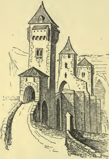
Fig. 20.—Fortified Bridge, from Valentré to Cahors (1308).
