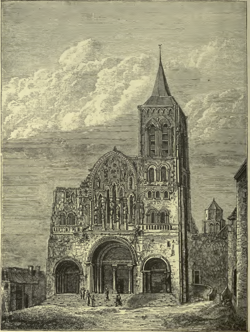
Fig. 105.—Façade of the Abbey Church of the Magdalen, as it now stands at Vézelay, where, in 1146, St. Bernard preached the Second Crusade (Twelfth Century).
