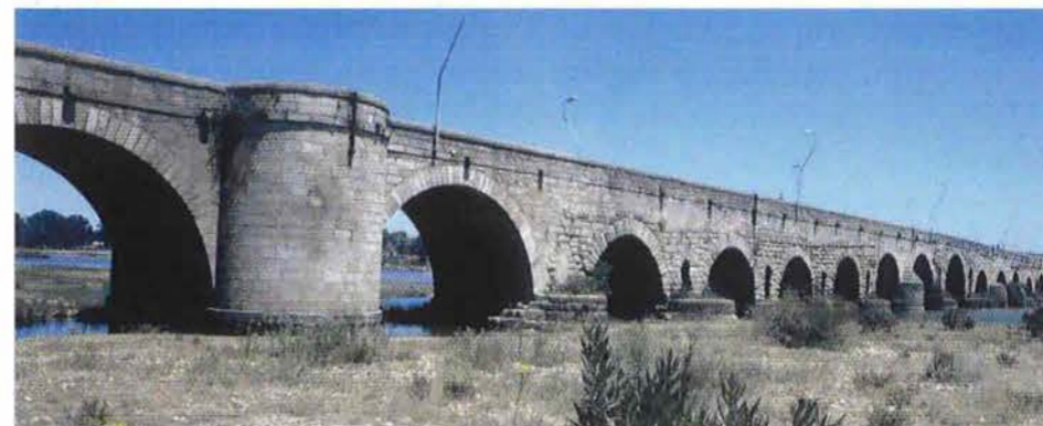
Merida Roman Bridge. The Romans were some of the earliest people to excel in bridge building, often using the circular arch to make their bridges strong. (© R. Sheridan/AAA Collection Ltd)
