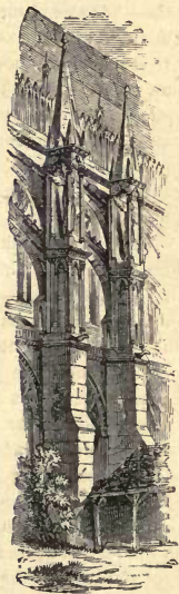
FIG. 17.—Flying buttresses weighted with pinnacles, from Rheims.
