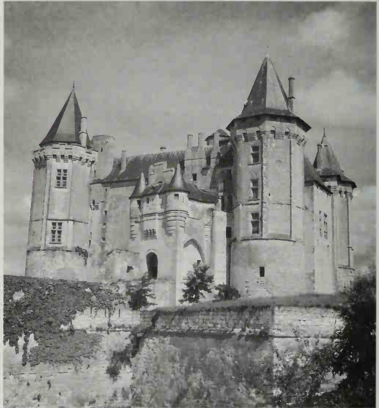
This view of Saumur Castle in France shows both smaller original windows (at top of gatehouse) and much larger windows added later (in round corner towers).
