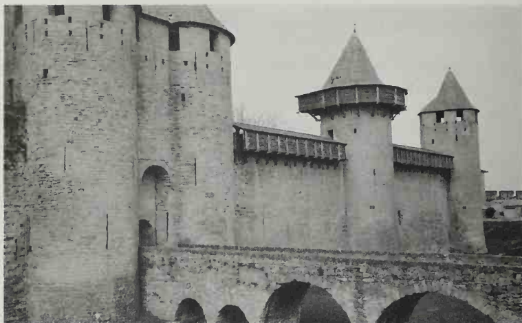
This twelfth-century French castle displays numerous arrow loops and square holes for attaching wooden hoardings.
