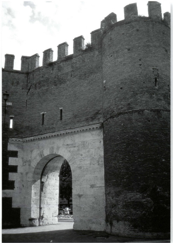
Exterior view of Porta Pinciana, looking south in Piazza Brasile. The round-fronted tower on the right was built onto this Type III gateway under Maxentius. (Author's collection)
