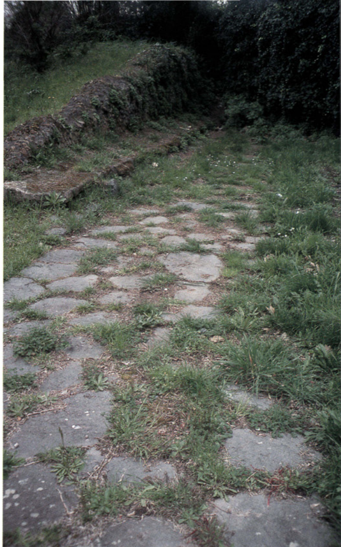
A close-up shot of Via Ardeatina, running south-east out of Porta Ardeatina, showing the agger or embankment, basalt metalling, and one of the gutters. (Author's collection)
