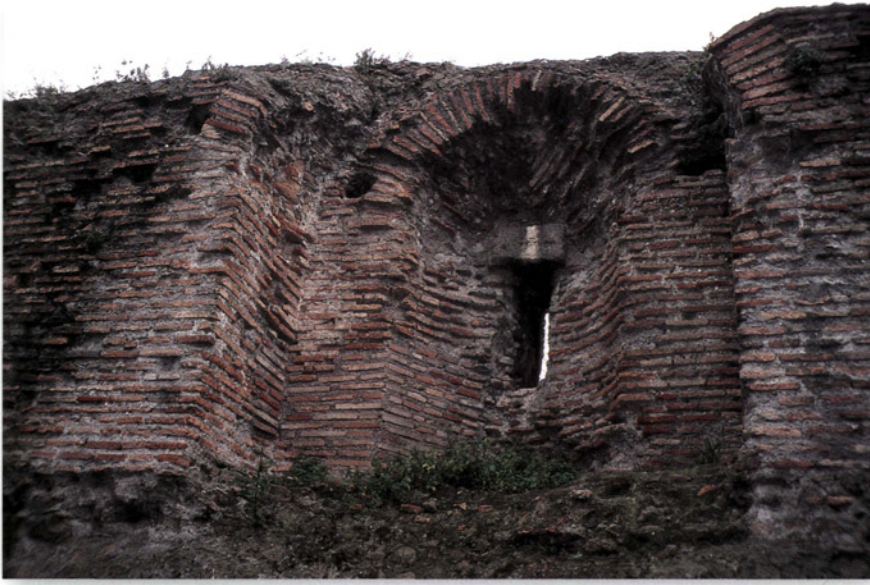
The brick-faced concrete construction on the interior of a tower in Viale Giotte. Once properly set, it created a homogeneous mass that was less vulnerable to collapse than dry stone construction. (Author's collection)
