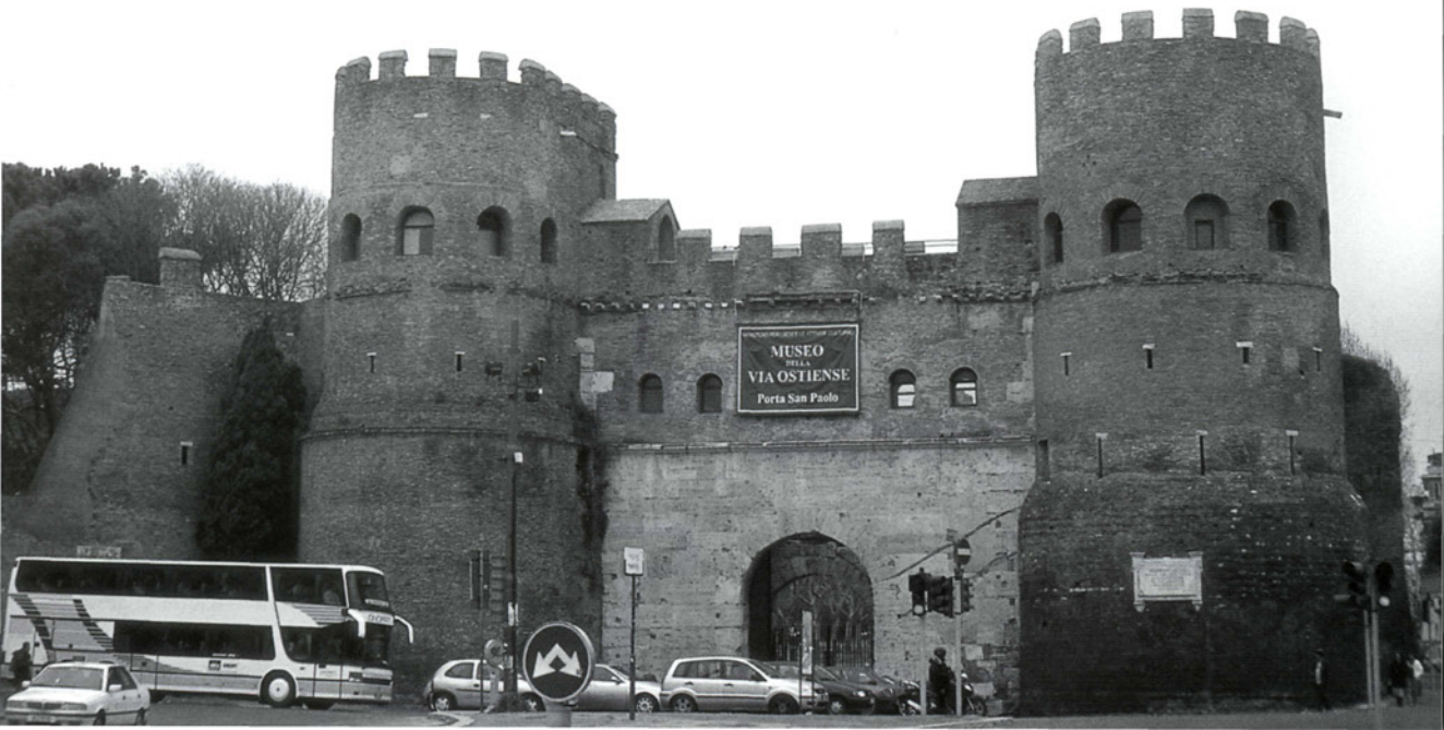
An exterior view of Porta Ostiensis East, looking north-north-west in Piazzale Ostiense. Like Porta Appia, this was a Type I gateway and thus served a main axial road into Rome. (Author's collection)
