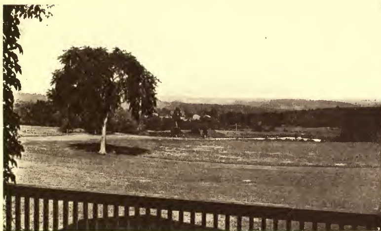
VIEW FROM REAR PIAZZA OF THE BROOKS HOUSE
