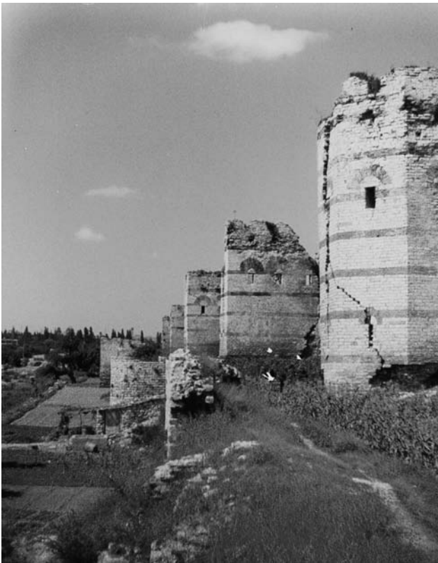
Figure 2 The walls of Constantinople, often repaired but basically late Roman in design and technique
