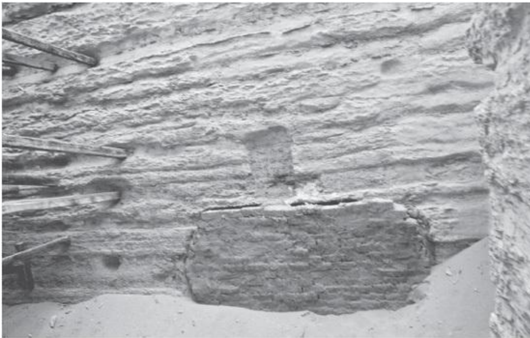
Figure 14.8. One of several blocked-up entrances
