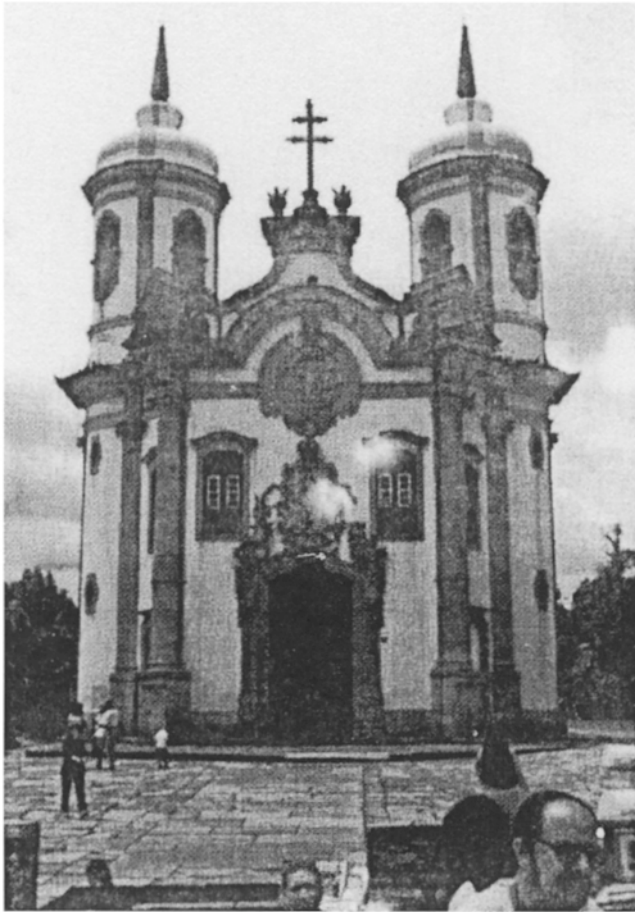
Figure 3.5 St Francis of Assisi Church building, Ouro Preto, Minas Gerais, Brazil; eighteenth century (Pifano 1996:131–4).
