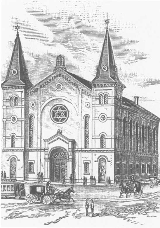
Figure 17.3 Adath (Temple) Israel's first purpose-built synagogue, 1885, was the source of the widespread Rundbogenstil synagogue style in Boston (see Figure 17.1, 2b). Main elements copied in other synagogues include the rounded windows and doors, especially the narrow windows flanking the front door, the round window with the Jewish star, the large high arch above it, and the gable end topped by the Ten Commandments. The tall Bavarian church steeples topped by Jewish stars were not copied (Kaufman 1995:176, 182). Photograph courtesy of the American Jewish Historical Society.
