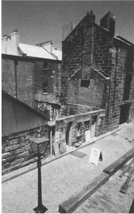
Figure 16.13 Looking to south east, over Kendall Lane and the archaeological site, prior to rebuilding, 1991. The profile of the 1844 cottage was preserved in the wall of the ‘Coachhouse’, built adjoining and slightly around the earlier structure. The wall fronting the lane is largely original (photograph by the author).
