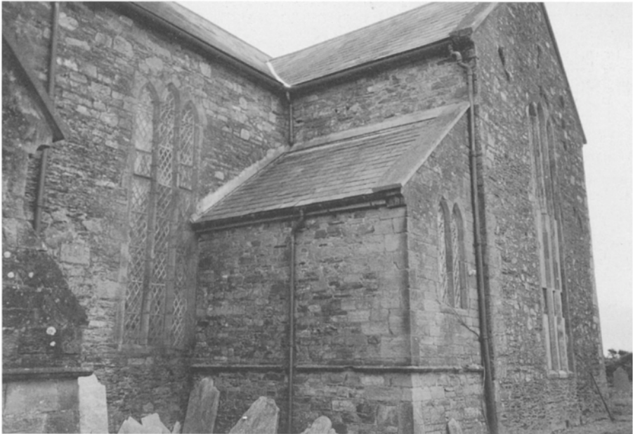
Figure 10.8 Christ Church, Bandon, south nave and transept, with a later chapel blocking an original window. Note the change of masonry two-thirds up the walls; below are coarse, thin slabs horizontally laid in the seventeenth century; above is uneven ashlar block construction, contemporary with the insertion of Gothic style windows in the eighteenth century (photo, E.Klingelhofer).
