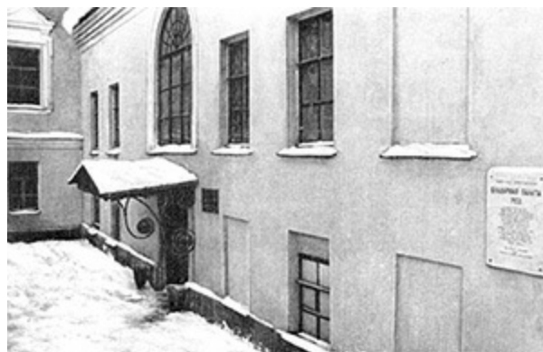
Fig. 3.32. The small building inside the citadel of the modern Novgorod upon River
