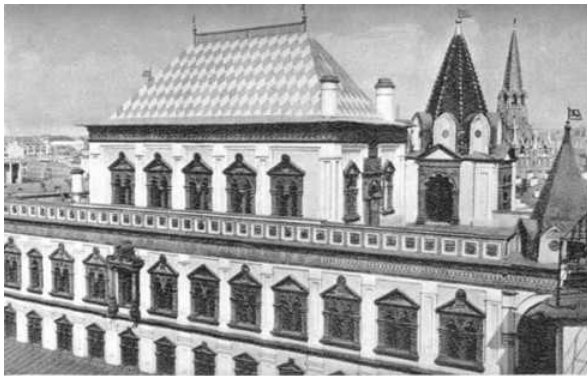
Top part of the building as seen from the outside
