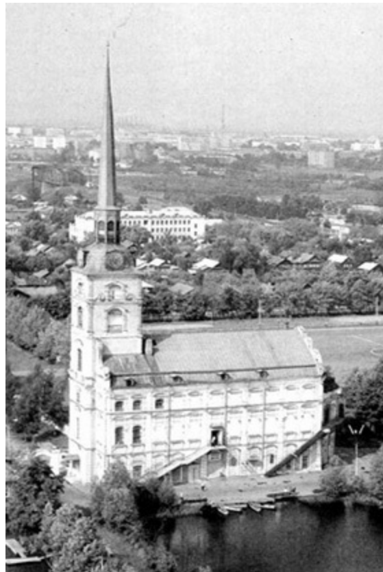
Fig. 14.227. The Gothic Cathedral of Peter and Paul in Yaroslavl, built in the Old Russian style of the Horde. We see a spire, a gable roof and a first floor entrance.
