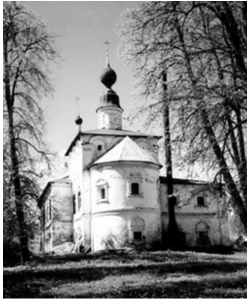
Fig. 14.225. The Church of Presentation, Nikolo-Ouleimenskiy Monastery, Ouglich. Eastern view. A more recent square block topped by a cylinder and also characterised by a semicircular altar part was adjoined to the old building in some later epoch. Photograph taken in 2000.
