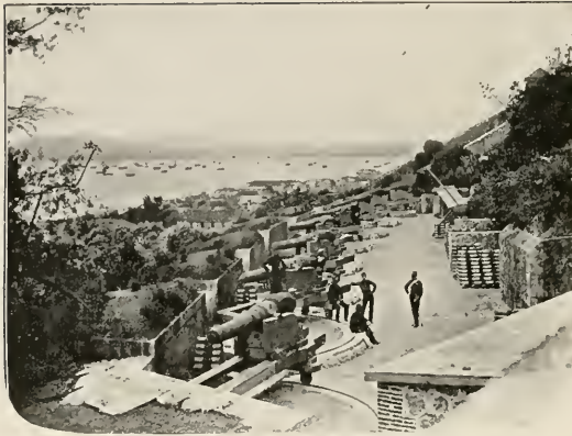
ONE OF MANY BATTERIES.
