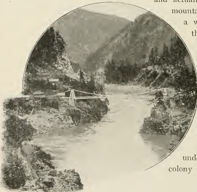
CARIEOU ROAD BRIDGE, BRITISH COLUMBIA.
