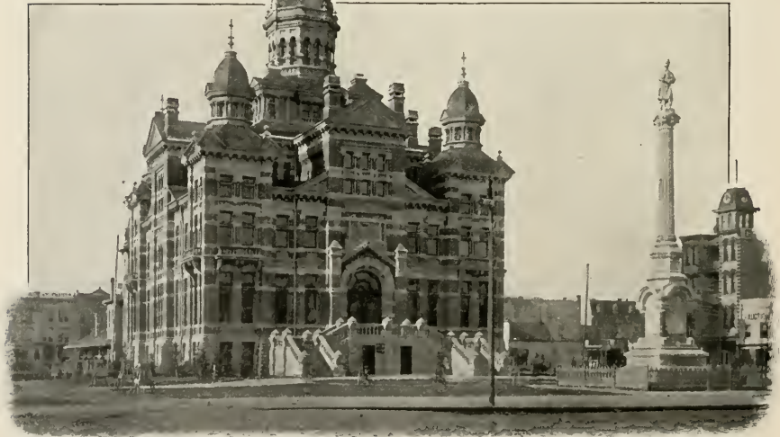
CITY HALL AND VOLUNTEER MONUMENT, WINNIPEG.
