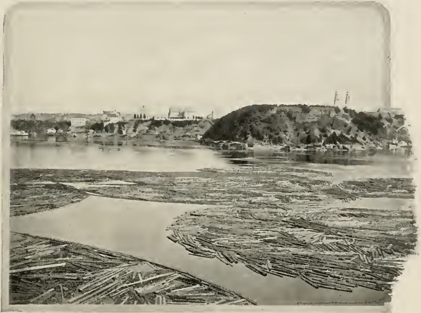
TIMBER BOOMS, OTTAWA RIVER.
