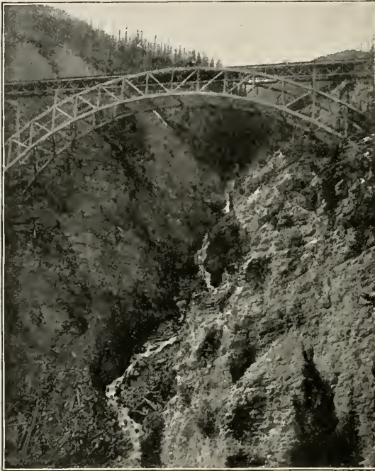
STONY CREEK BRIDGE.
