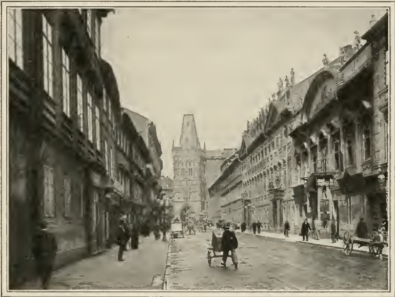
A DISTANT VIEW OF THE POWDER TOWER.
