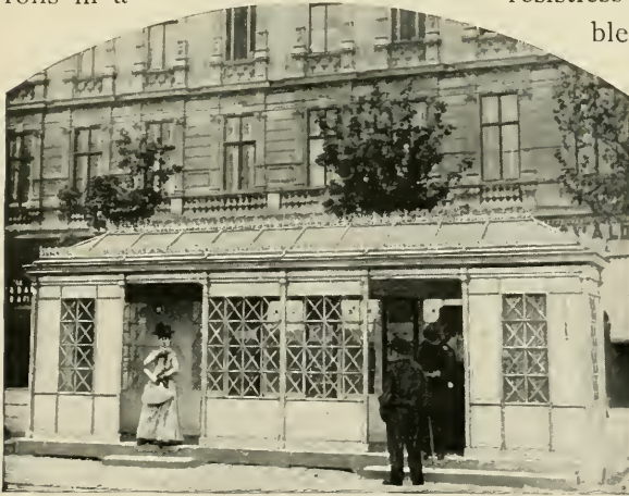
A STREET CAR STATION.
