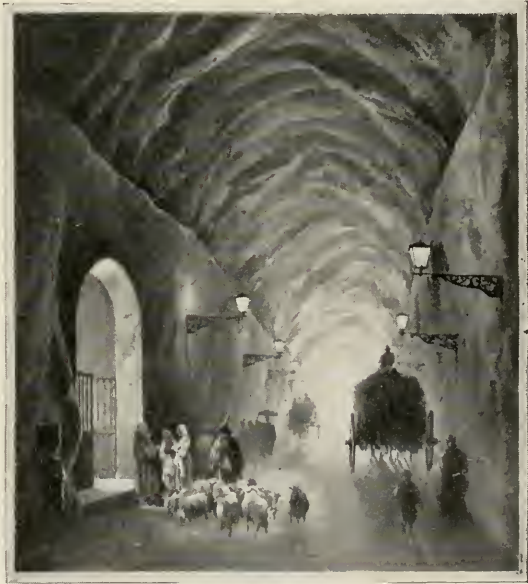
THE OLD TUNNEL.
