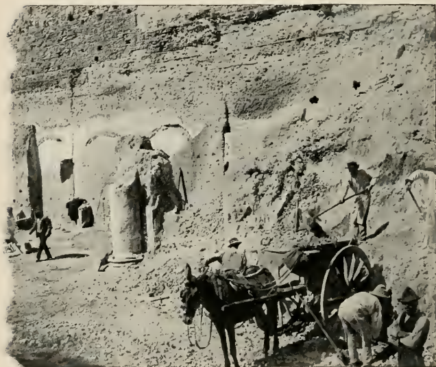
PROCESS OF EXCAVATION.
