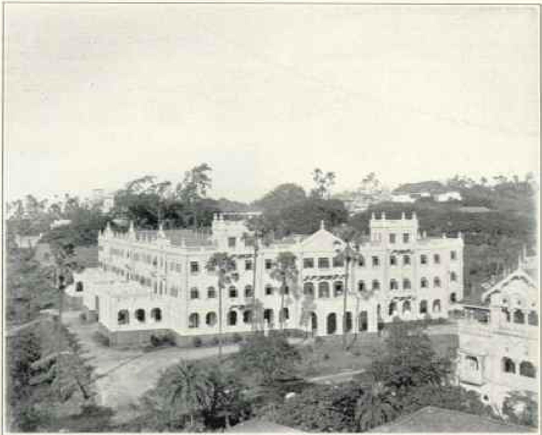
The Framjee Dinshaw Petit Parsee Sanitorium
