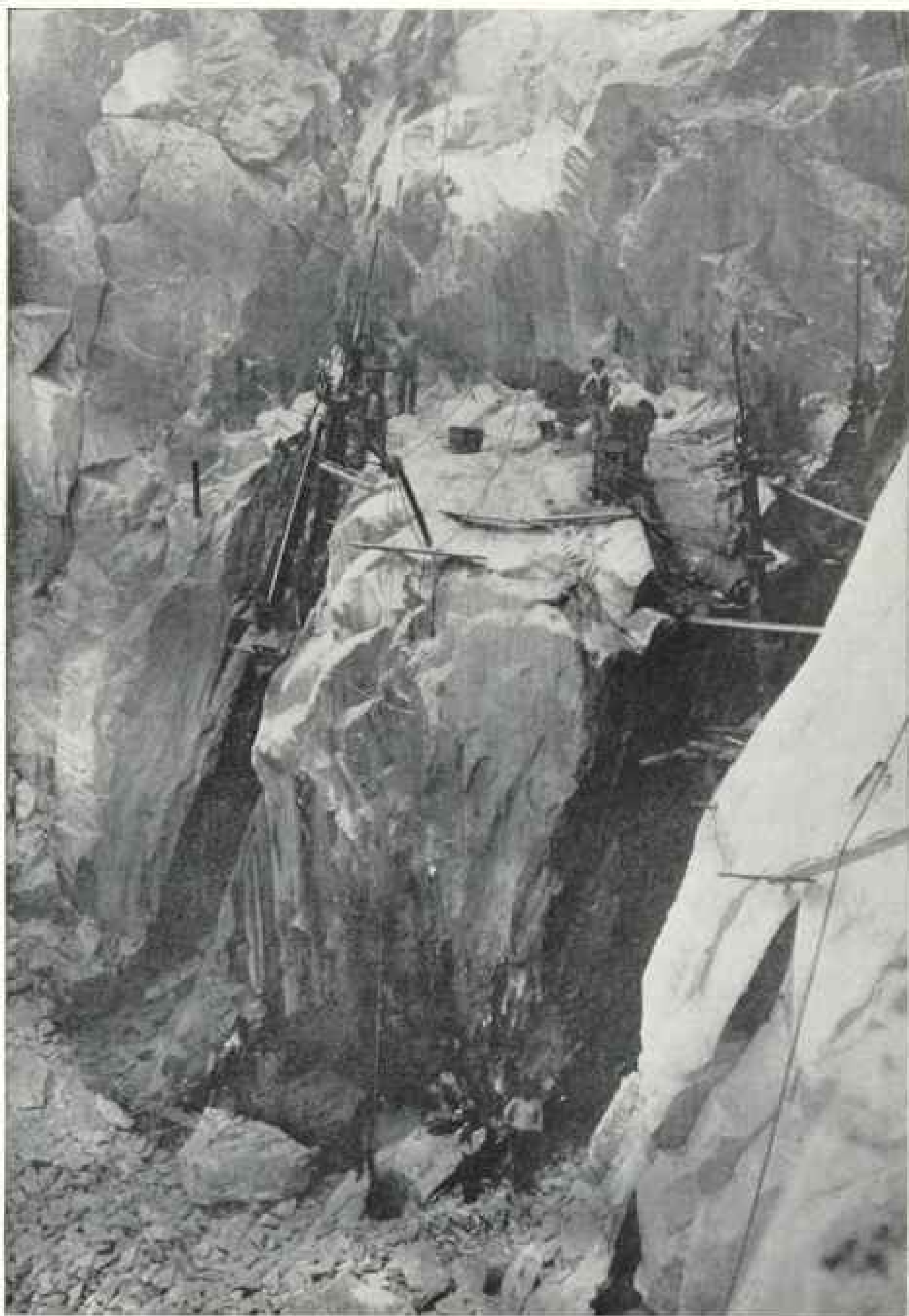
A MARBLE QUARRY, CARRARA: PREPARATION OF A CHARGE OF DYNAMITE TO DETACH A BLOCK OF MARBLE FROM THE MOUNTAIN SIDE
