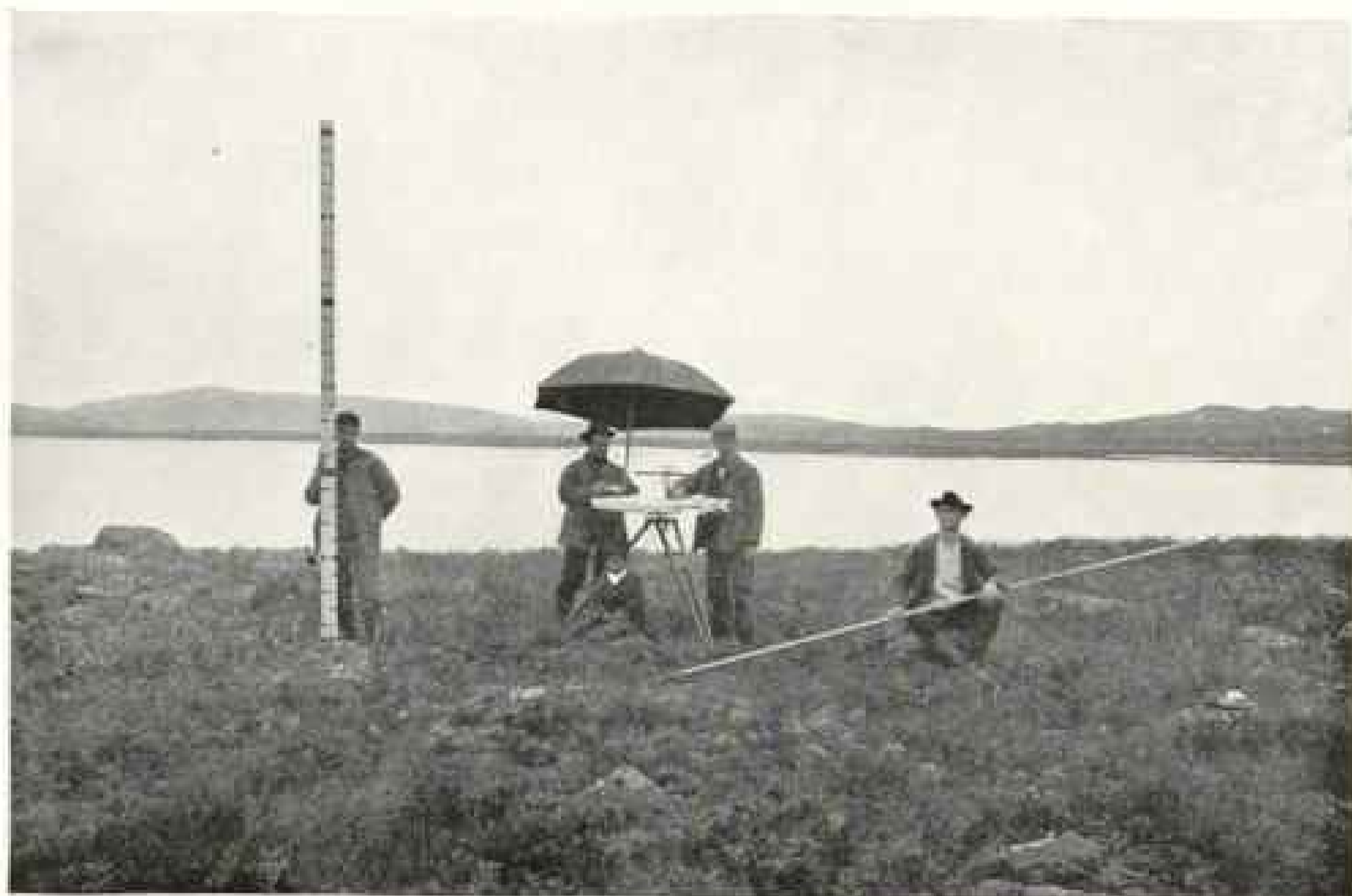
A PLANE-TABLE SURVEYOR MAPPING A SECTION OF SHORE-LINE
